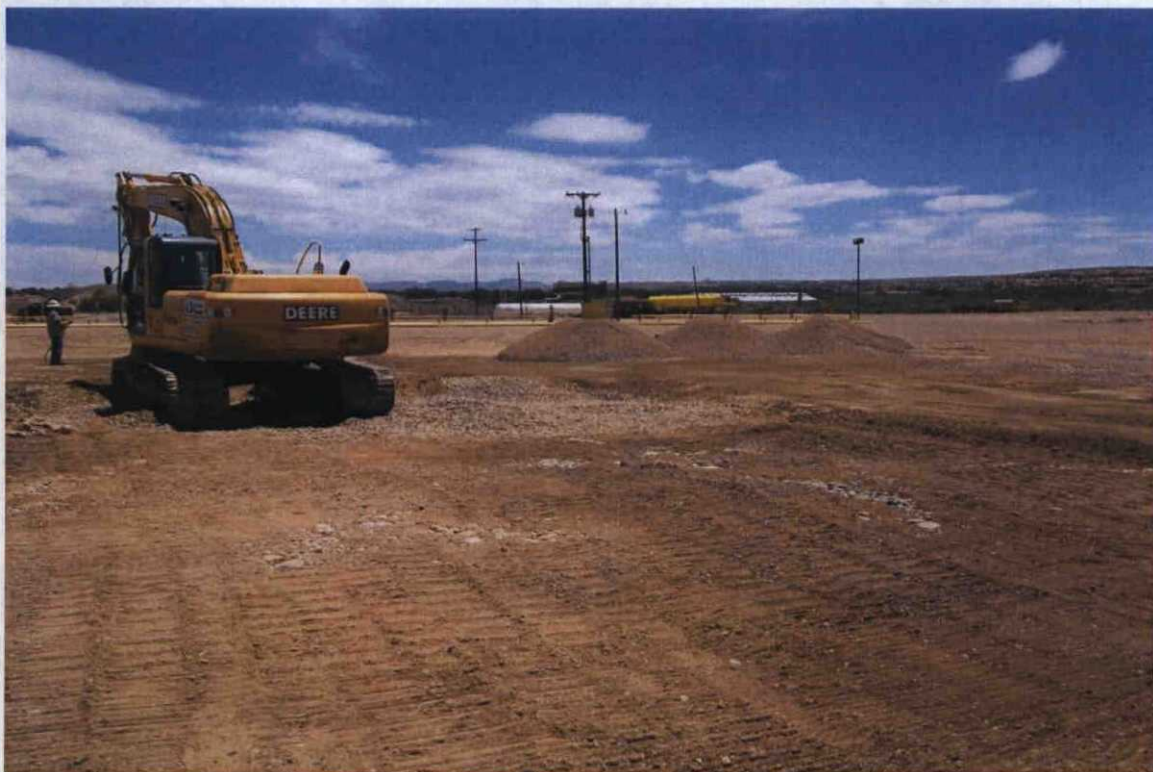
Photo 32: View of backfilling and compaction activities.
