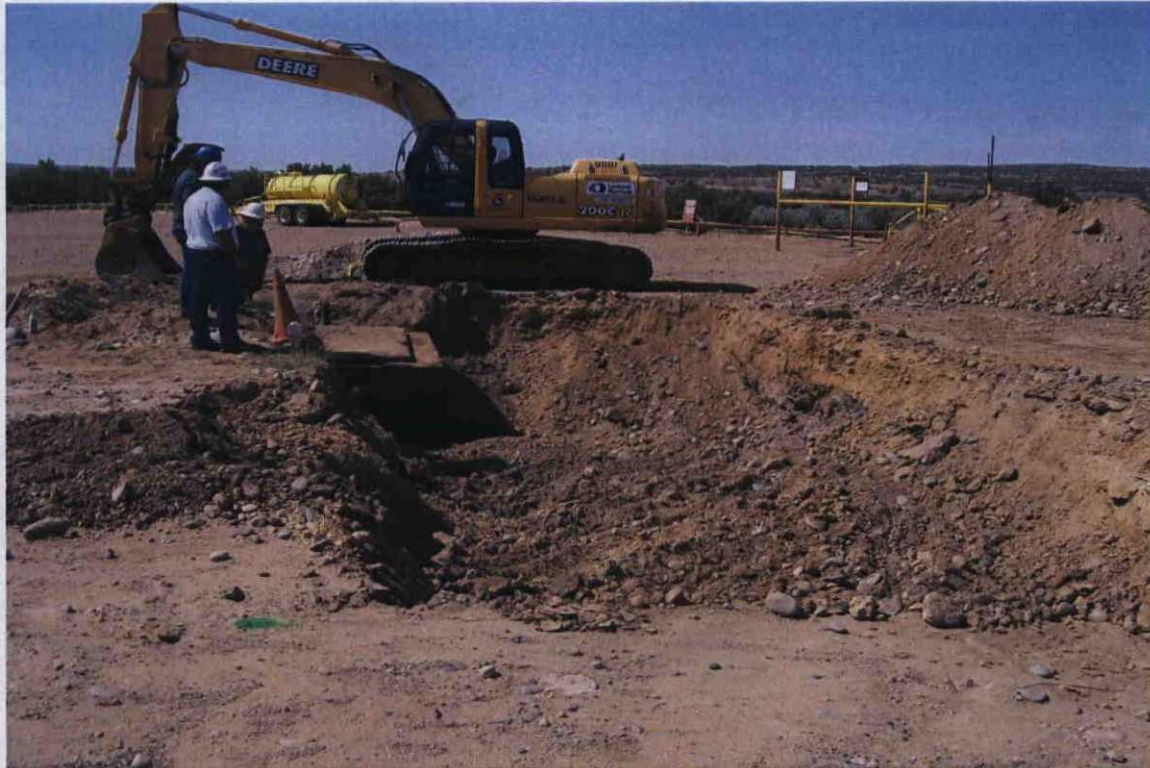
Photo 3: View of the excavation around the wash tank.
