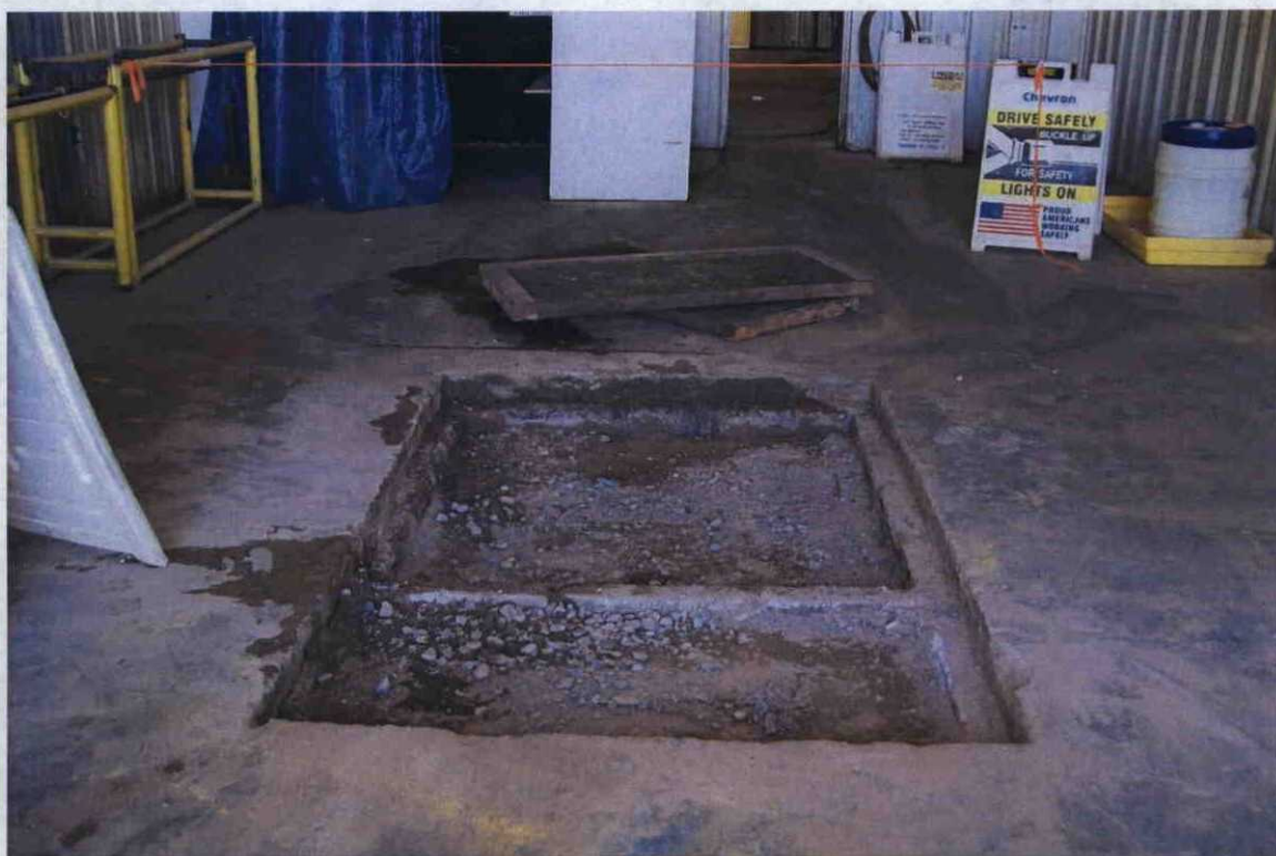
Photo 42: View of backfilling and compaction activities of the wash bay sumps.
