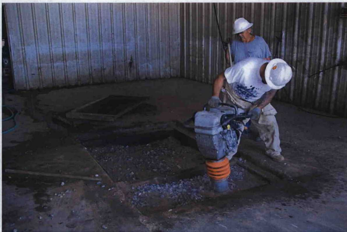
Photo 40: View of backfilling and compaction activities of the wash bay sumps.
