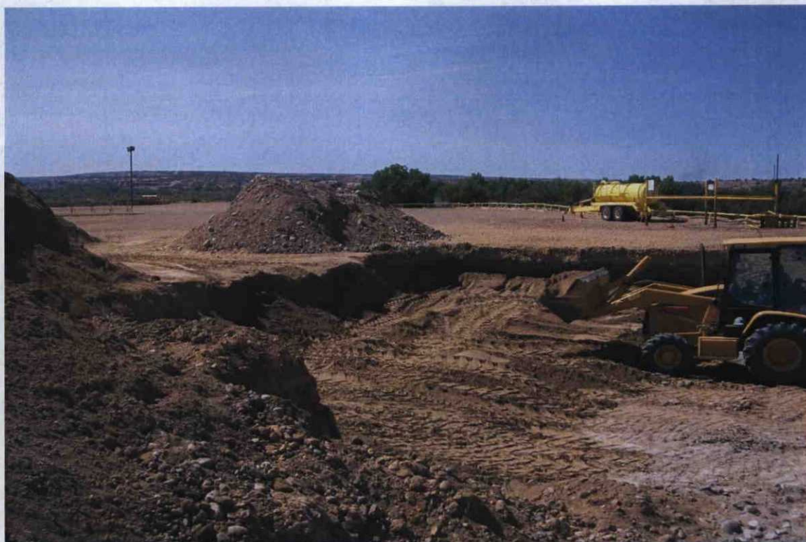
Photo 21: View of backfilling activities on the east side of the excavation.
