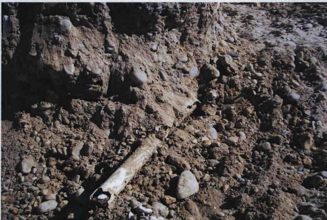
Photo 10: View of a leach line discovered during excavation activities on the northwest side.
