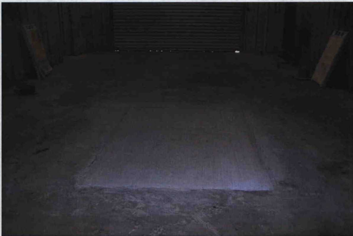
Photo 44: View of wash bay sumps after concrete completions.
