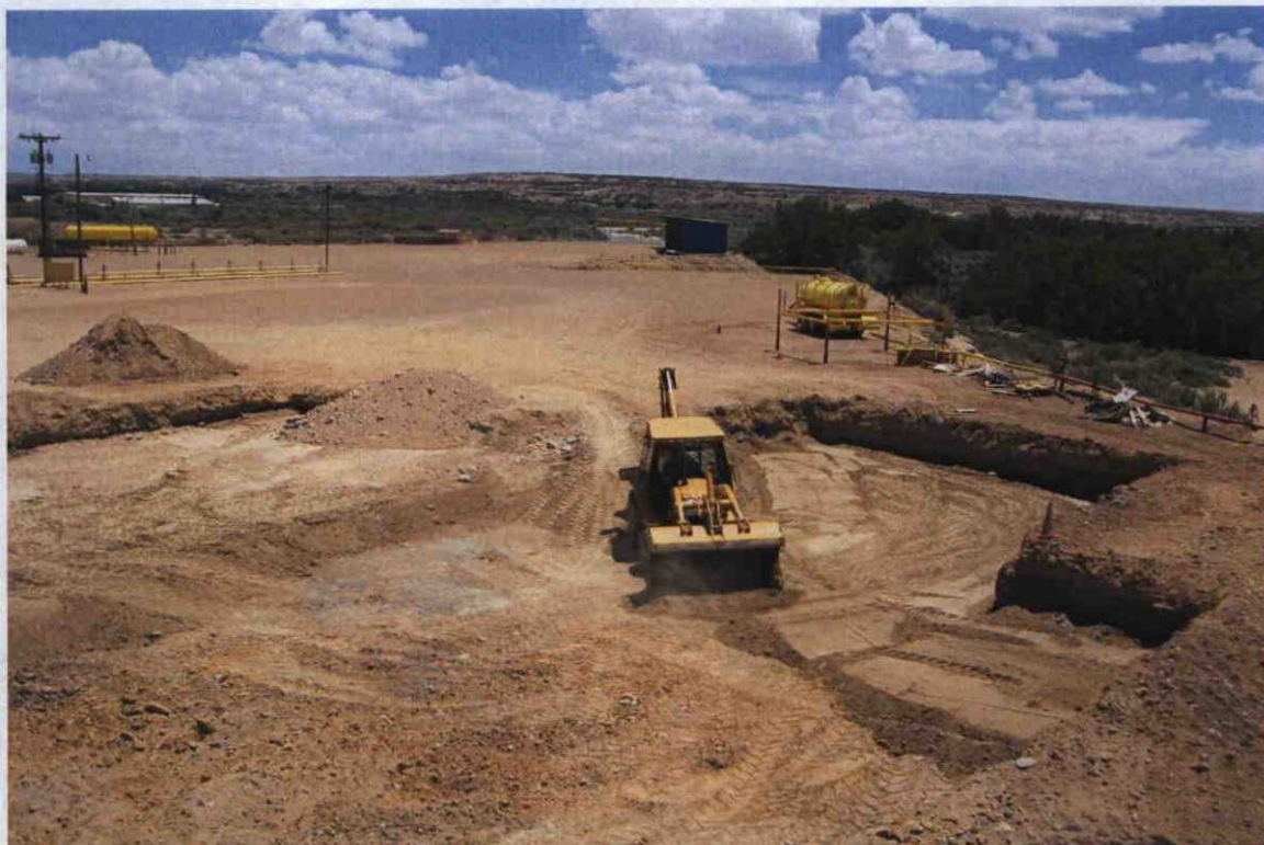
Photo 24: View of backfilling activities of the excavation.
