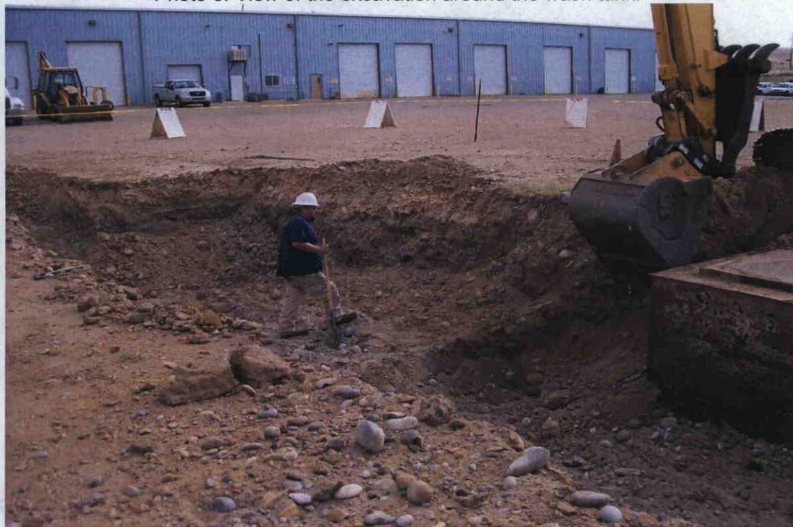
Photo 4: View of the excavation around the wash tank.
