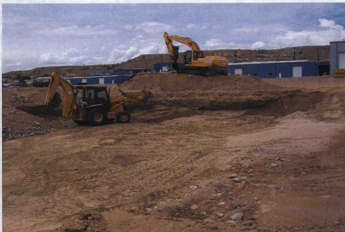
Photo 26: View of backfilling activities of the excavation.
