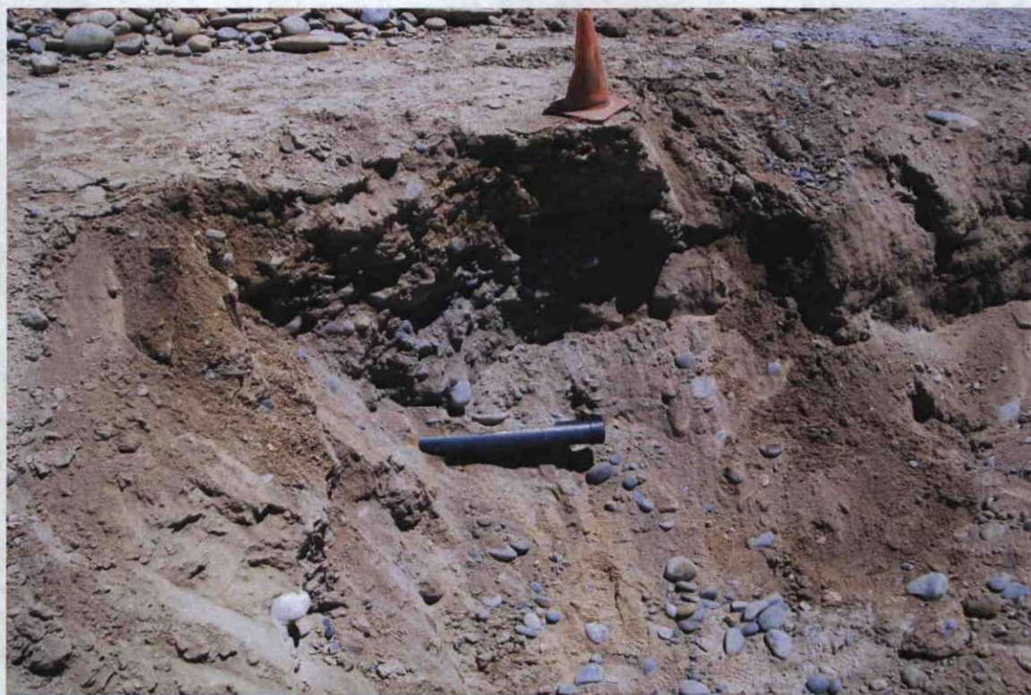
Photo 29: View of capped discharge line from the wash bays.
