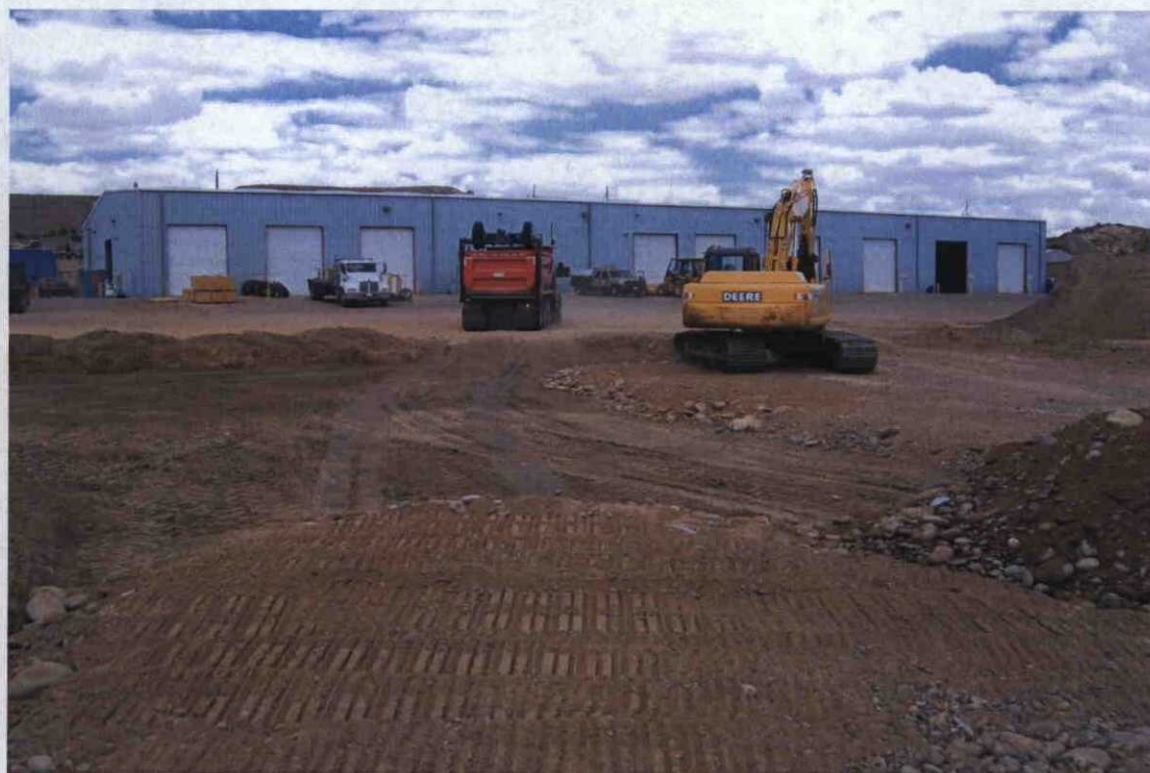
Photo 30: View of backfilling and compaction activities.
