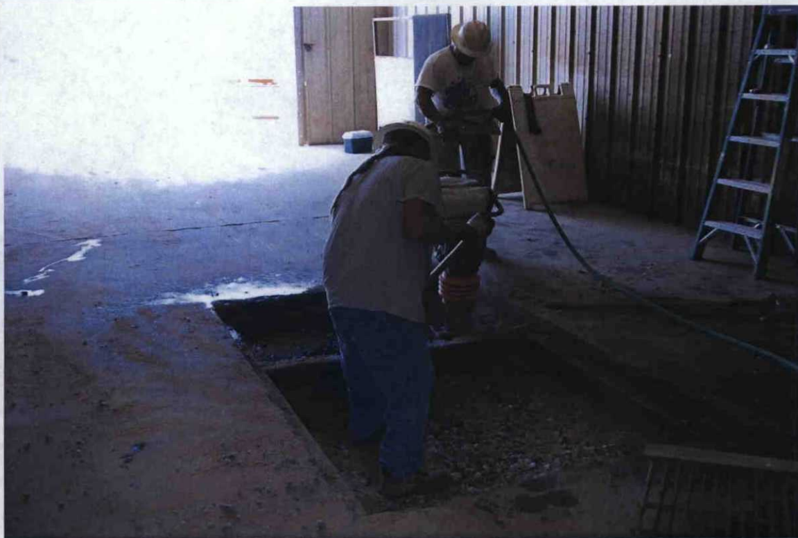
Photo 41: View of backfilling and compaction activities of the wash bay sumps.
