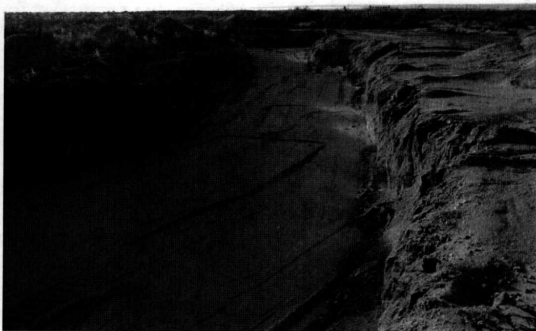
Photograph No. 6 – Looking easterly at final excavation and layer of cushion top soil across bottom for 40-mil polyethylene liner
