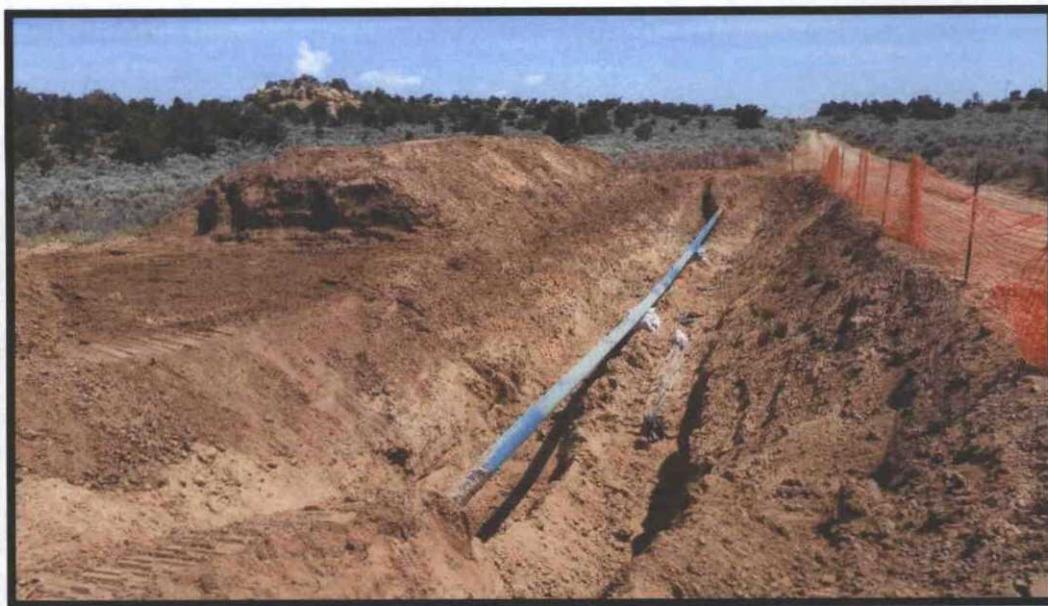
Photo 3: Deeper base section visible beneath repair, this area was excavated to 9 ft BGS.
