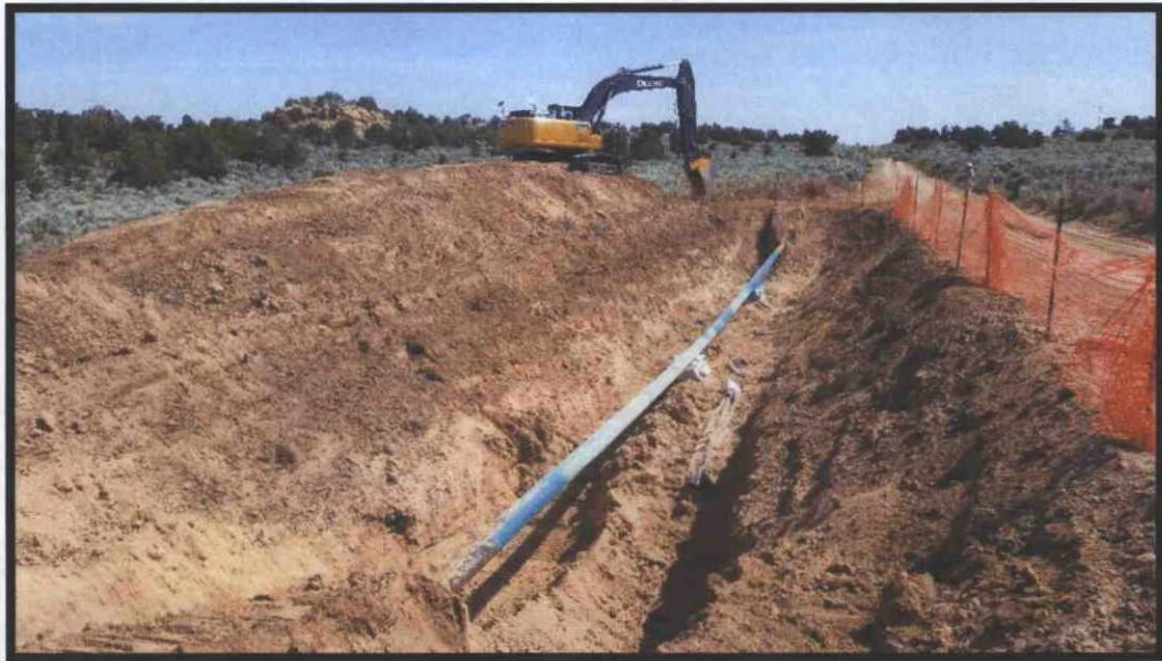
Photo 2: Track mounted excavator on site during sampling, final excavation extent pictured. Repair visible in foreground.
