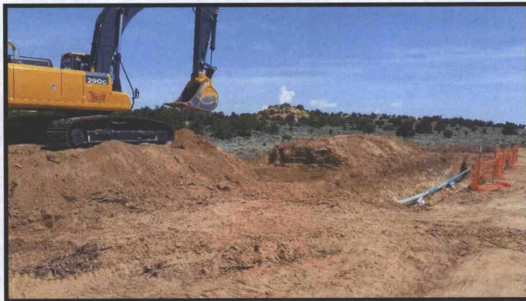
Photo 4: Track mounted excavator segregating stockpiles. The pile in the background (north) was sampled for use as backfill material.
