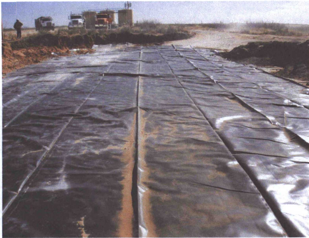
Installation of liner after excavation is backfilled to 4'
