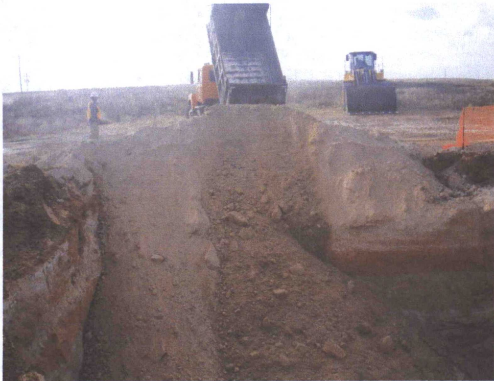
Backfilling with clean material
