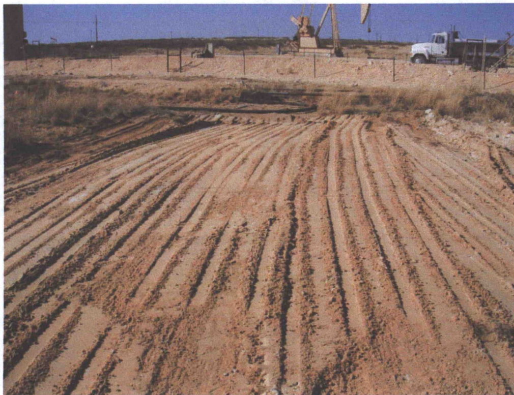
After liner was installed and clean material backfilled to surface grade
