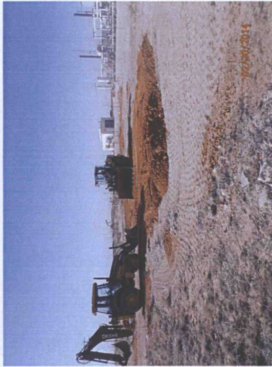
Backfilling scraped area with clay, facing north
