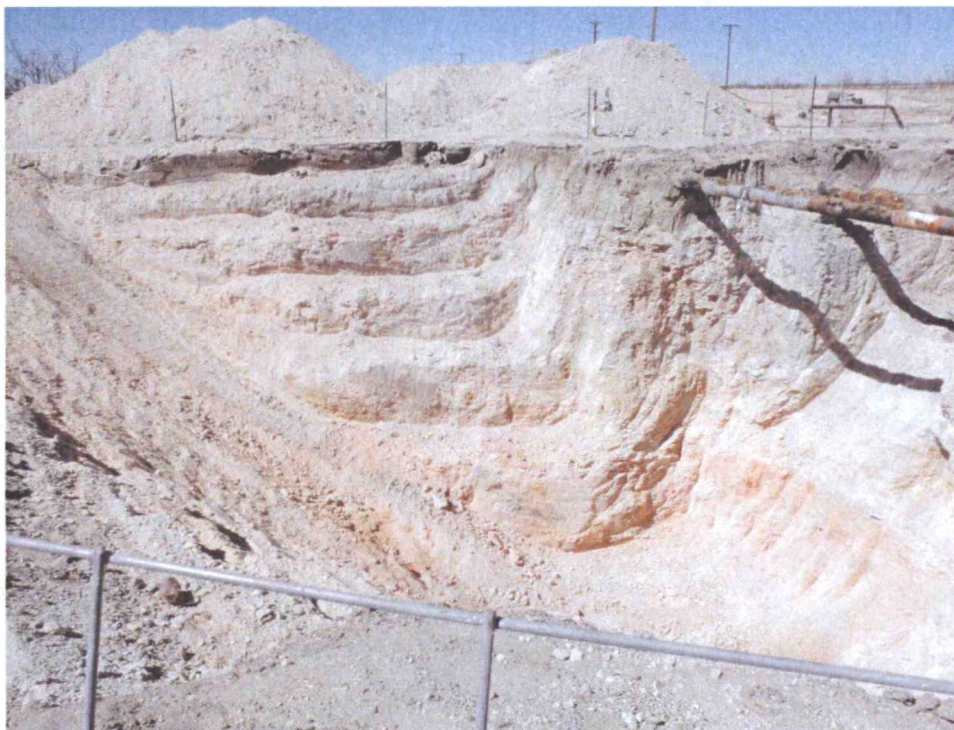
West Excavation after Benching Viewing West, March 2, 2011
