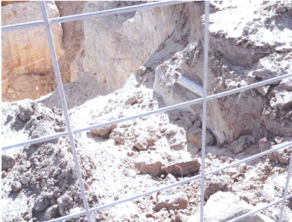
Produced Water (PVC) Line Exposed on North Side of West Excavation, March 2, 2011
