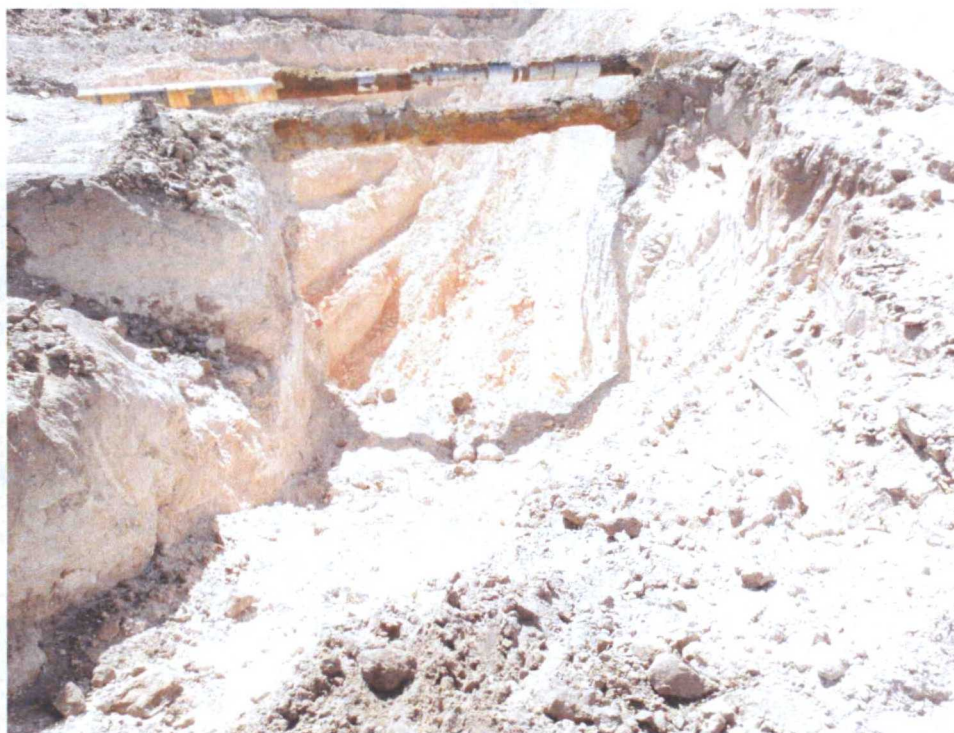
West Excavation after Benching Viewing South, March 2, 2011
