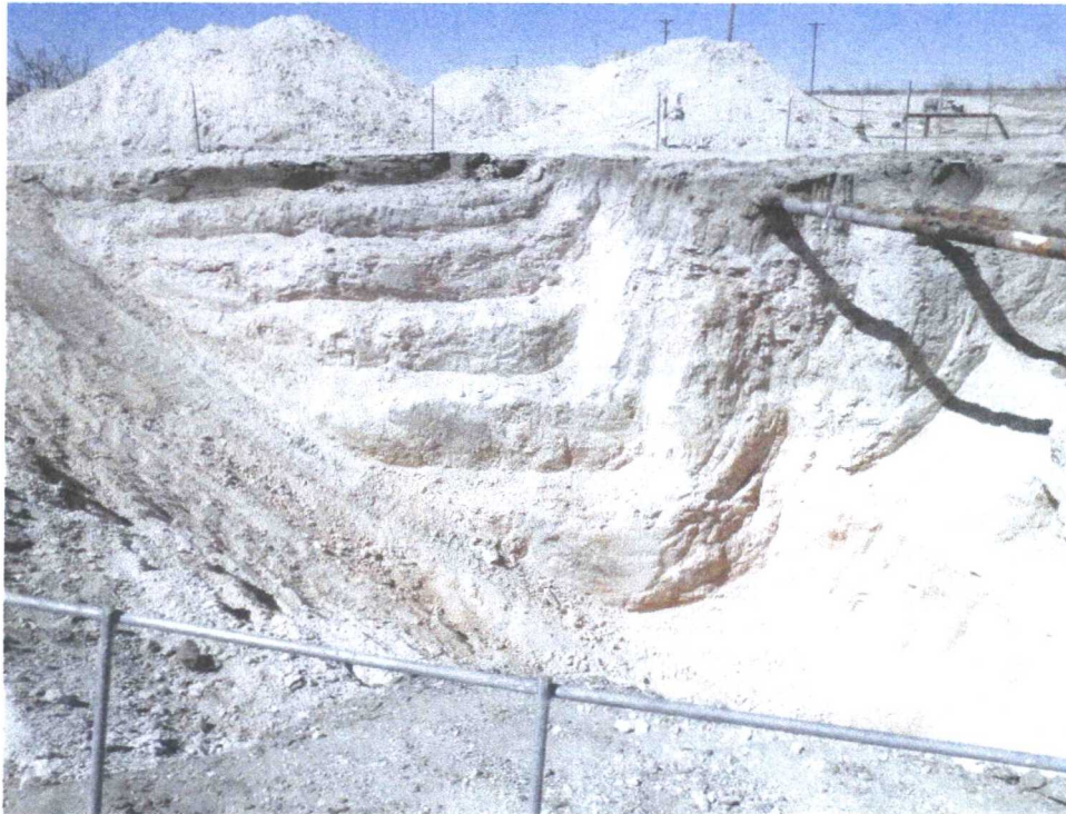
West Excavation after Benching Viewing West, March 2, 2011
