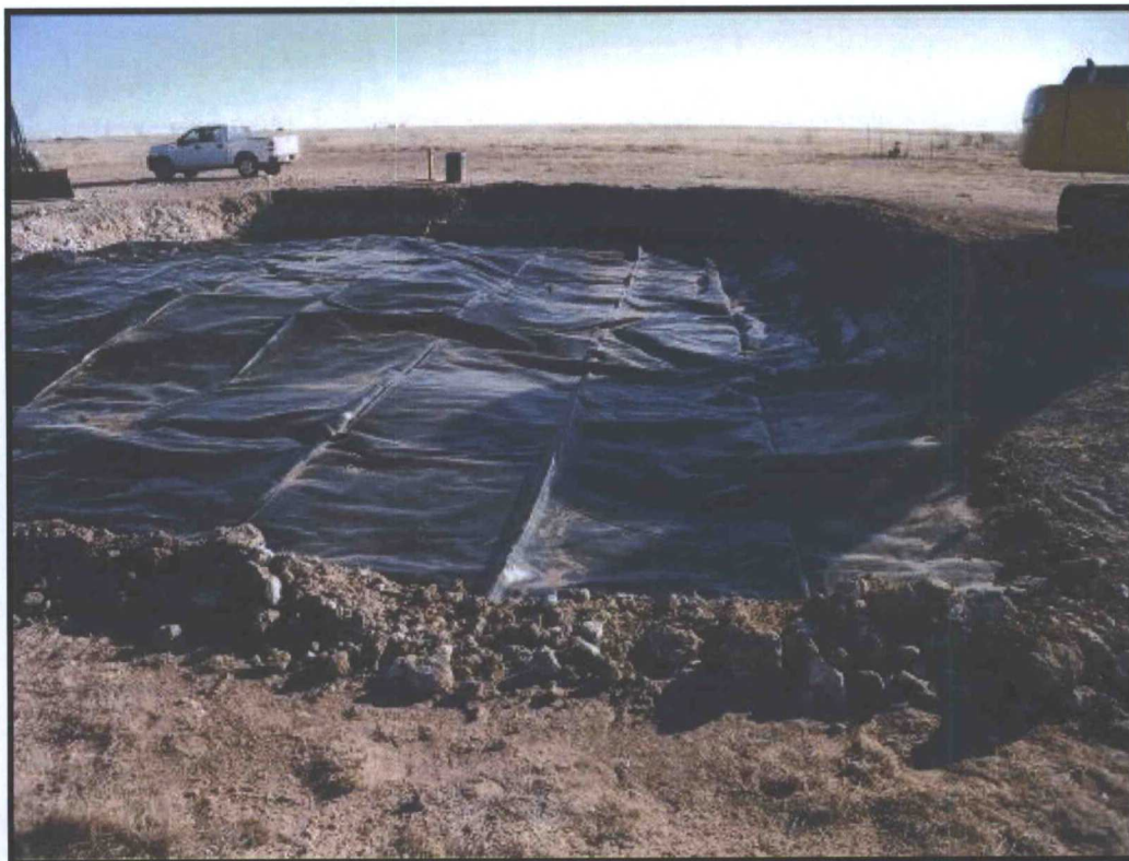
Southside excavation lined facing east
