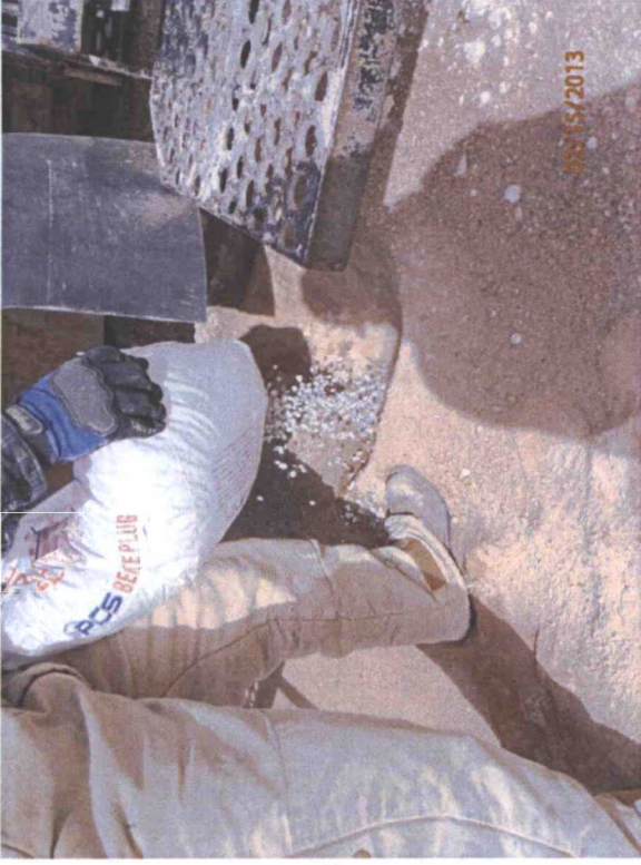
Plugging SB-1 in total with bentonite
