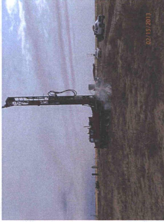
Installing Temp MW, facing east
