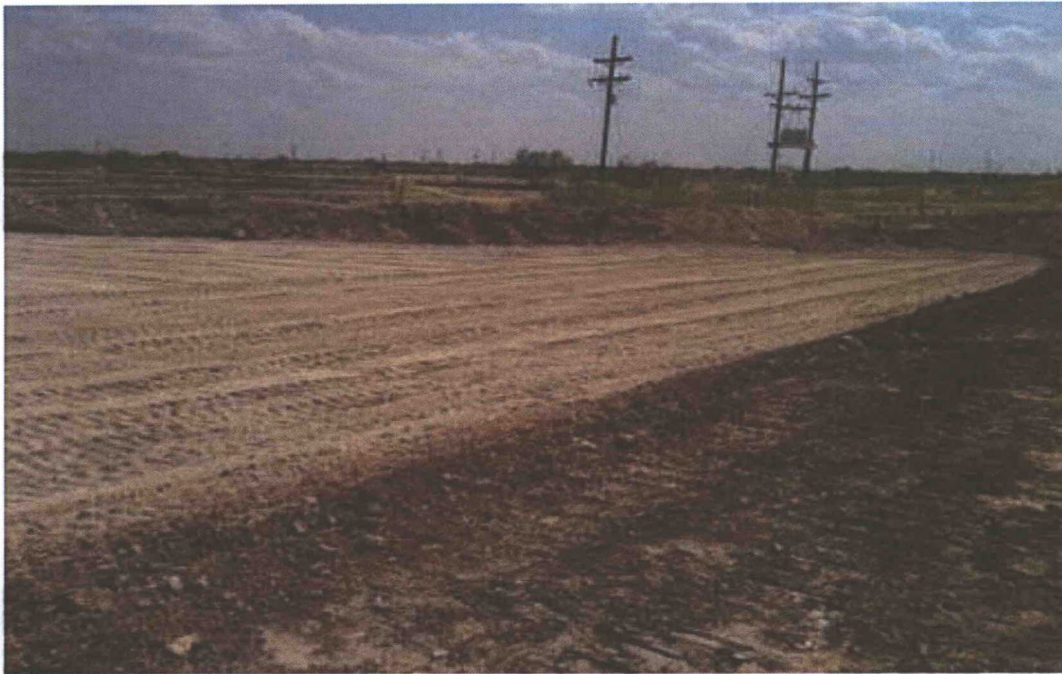
PHOTO 9: View of backfill ready for 20 mil poly liner installation facing northwest
