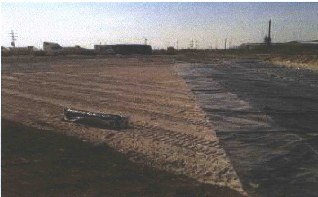
PHOTO 11: View of 20 mil poly liner installation facing southeast
