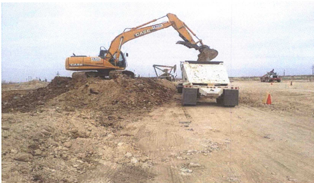
PHOTO 3: View of excavation/waste removal activities
