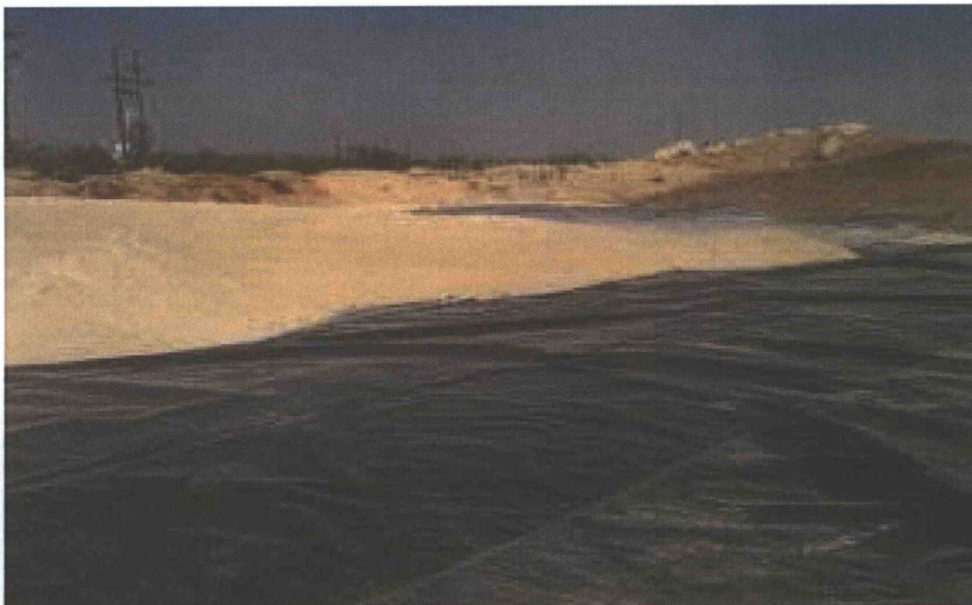
PHOTO 12: View of 20 mil poly liner installation/backfill facing northwest
