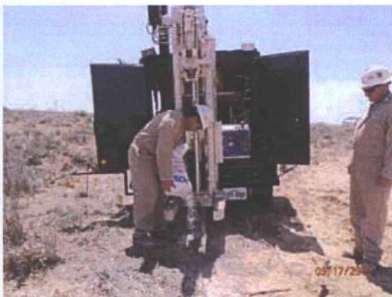
Plugging SB-2 in total with bentonite 5/17/12
