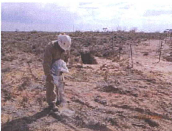
Plugging SB-10 in total with bentonite 5/17/12
