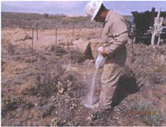
Plugging SB-7 in total with bentonite 5/17/12
