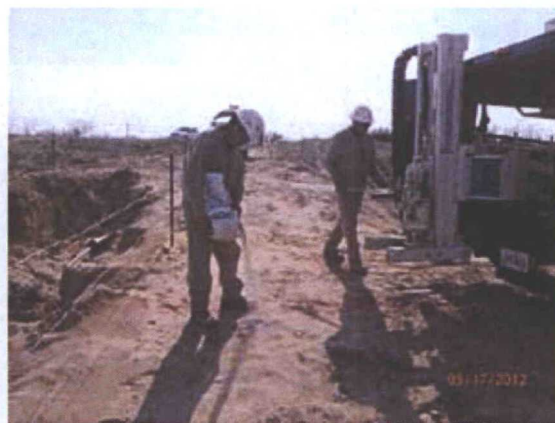
Plugging SB-11 in total with bentonite 5/17/12
