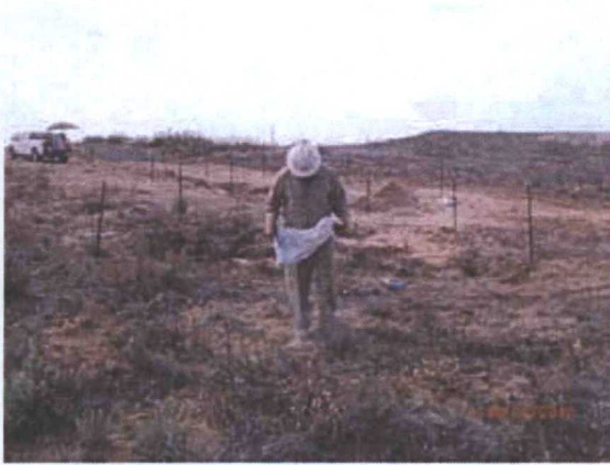
Plugging SB-9 in total with bentonite 5/17/12
