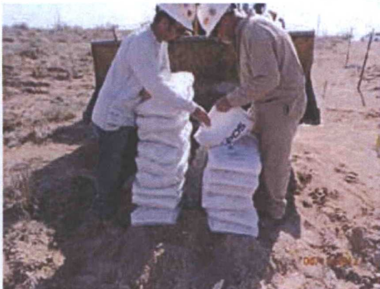
Plugging SB-13 in total with bentonite 6/11/12
