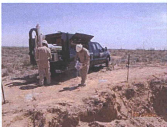
Plugging SB-4 in total with bentonite 5/17/12
