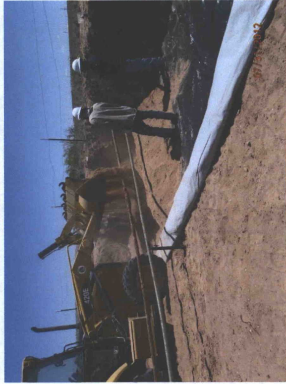
Backfilling above liner, facing north
