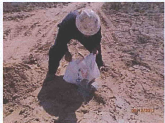
Plugging SB-14 in total with bentonite 6/12/12
