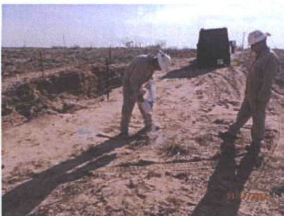
Plugging SB-12 in total with bentonite 5/17/12
