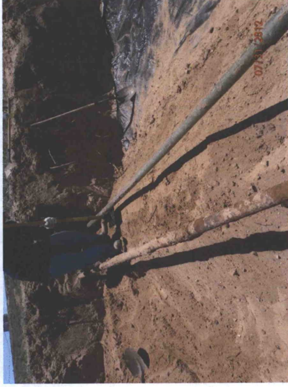
Packing soil under lines, facing east
