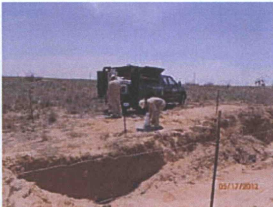
Plugging SB-1 in total with bentonite 5/17/12
