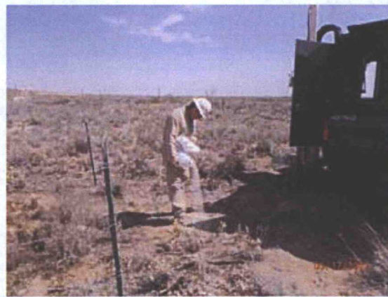
Plugging SB-6 in total with bentonite 5/17/12
