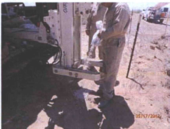
Plugging SB-3 in total with bentonite 5/17/12
