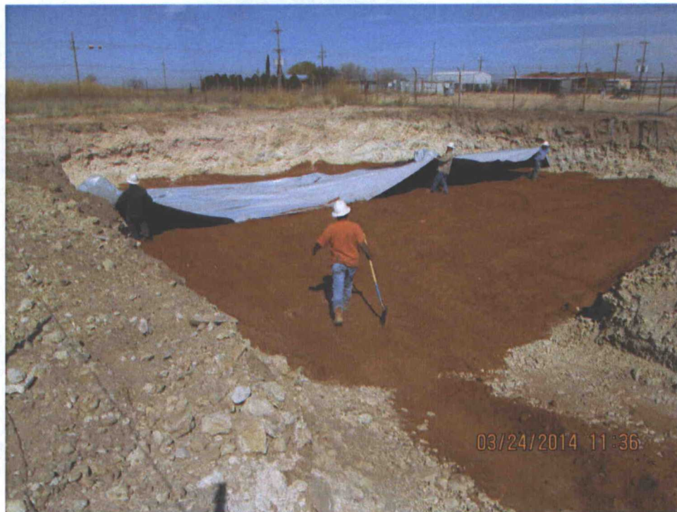
Pit #1 Liner Installation Viewing Northwest, March 24, 2014
