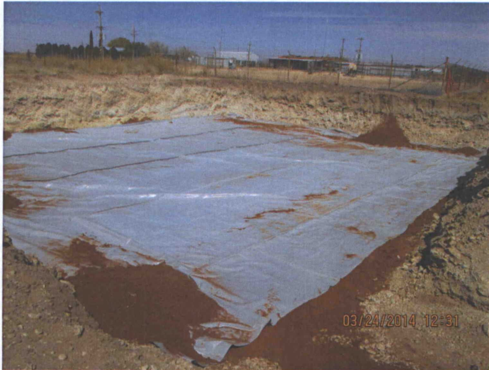
Pit #1 Liner Installation Viewing Northwest, March 24, 2014
