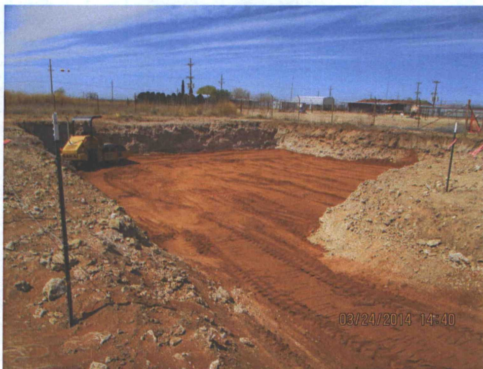
Pit #1 Liner Covered and Compacted Viewing Northwest, March 24, 2014
