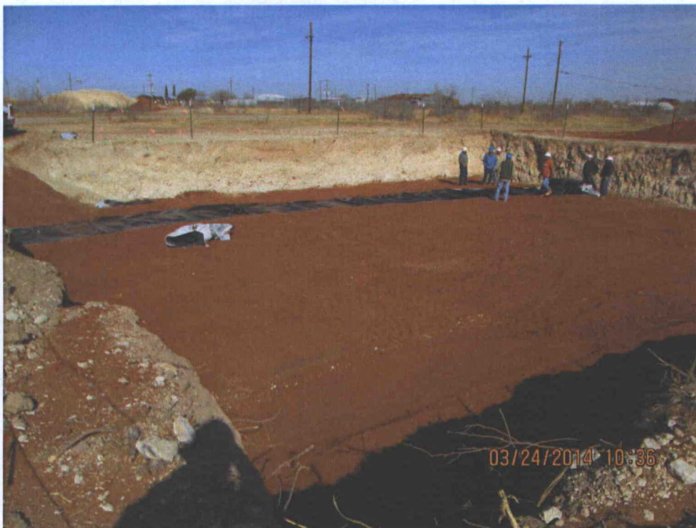
Pit #2 Liner Installation Viewing Northwest, March 24, 2014
