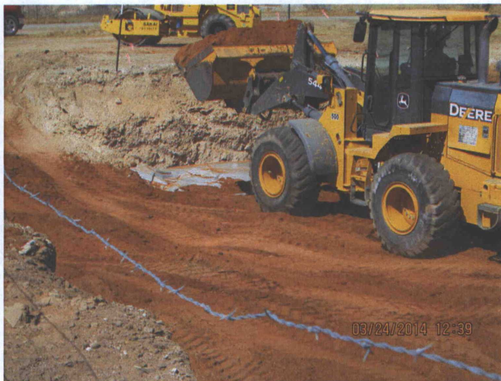
Pit #2 Covering Liner Viewing West, March 24, 2014
