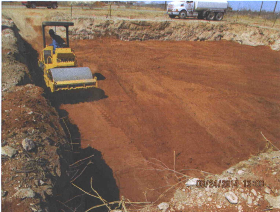
Pit #2 Compacting Cover Soil Viewing West, March 24, 2014
