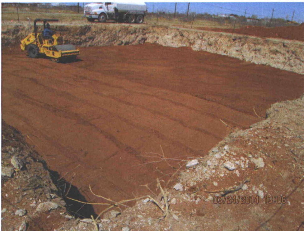
Pit #2 Compacting Cover Soil Viewing Northwest, March 24, 2014
