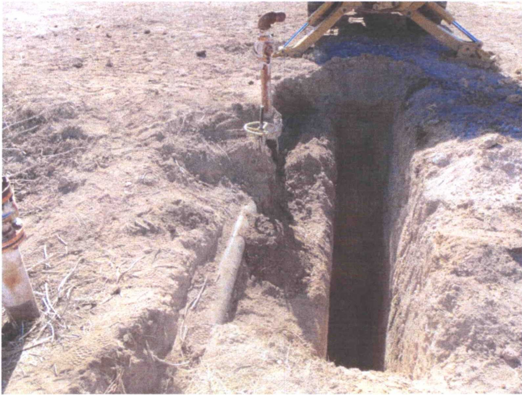
Photograph of the advancement of a delineation trench at the Line 2C 12" Release Site.
