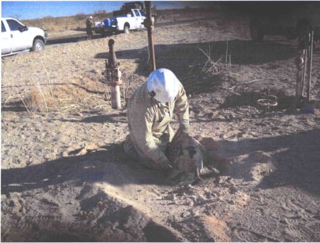
Photograph of the installation of bentonite plug in SB-1 at the Line 2C 12" Release Site.
