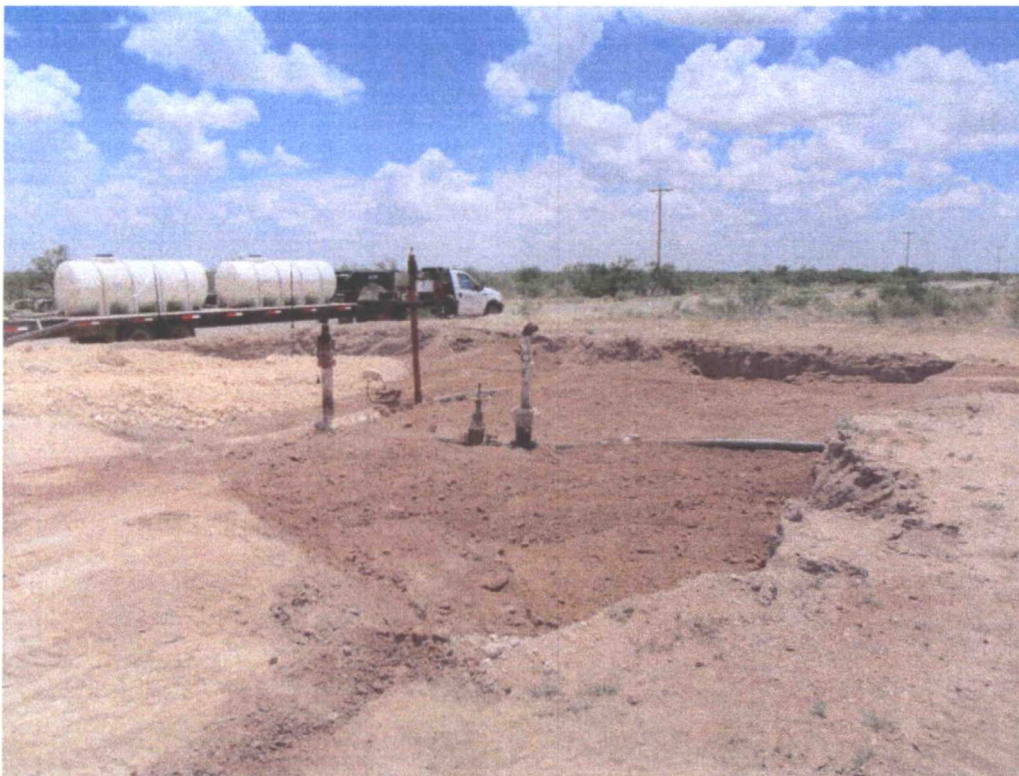
Photograph of installation of clay liner at the Line 2C 12" Release Site.
