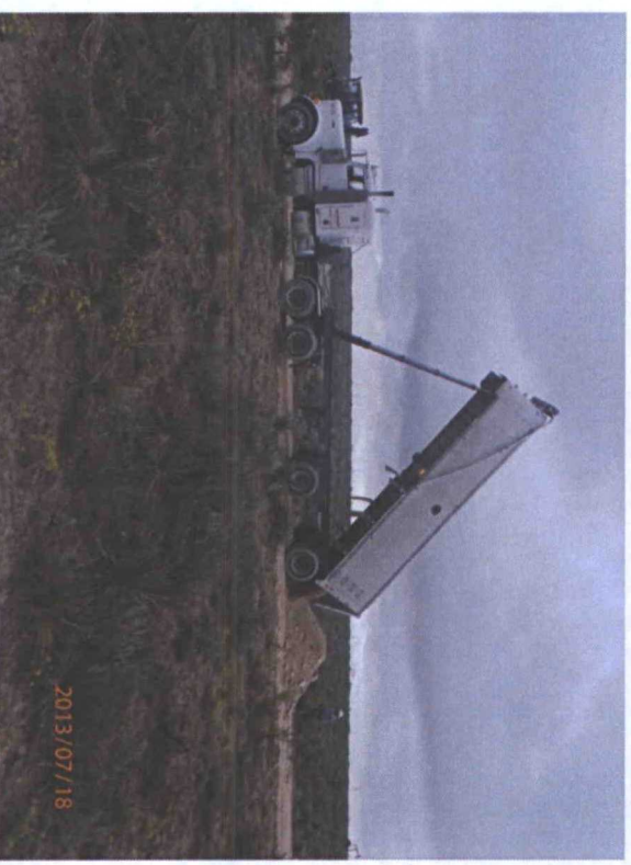
Import caliche to build surface for soil bore installations facing, west
