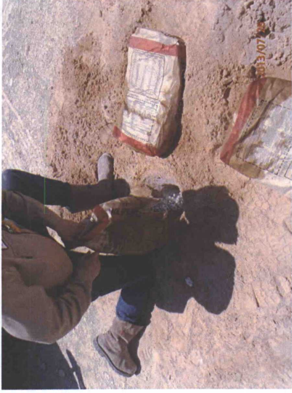
Plugging soil bore #1 in total with bentonite 7/26/13
