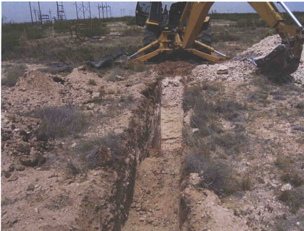
Photograph of delineation activities at the Eumont Tank Battery Remediation Site.
