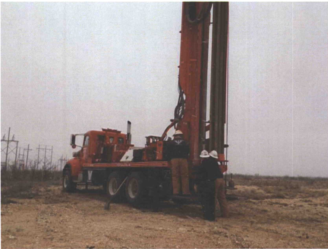
Photograph of the advancement of soil bores at the Eumont Tank Battery Remediation Site.
