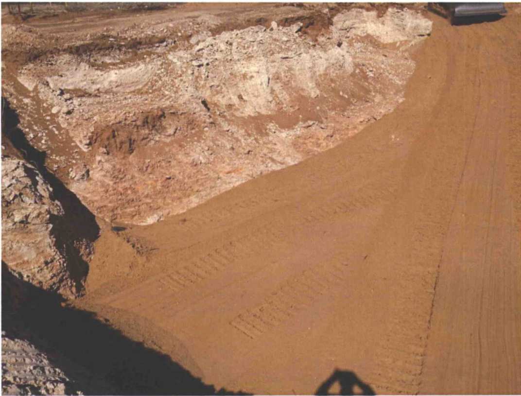
Photograph of the installation of pad sand at the Eumont Tank Battery Remediation Site.
