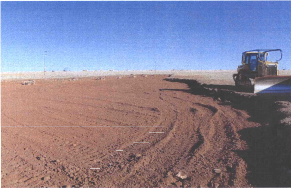
Denton SWD Historical Site #2 - Excavation (following installation of clay liner)
