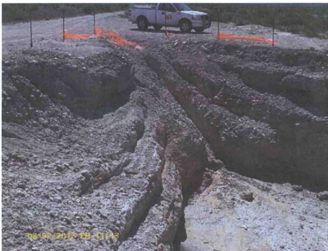
Photograph No. 1 – Looking southwesterly at former ingress/egress ramp and benched sidewalls of excavation
