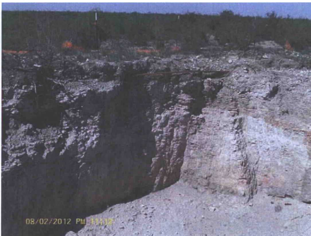
Photograph No. 2 – Looking northerly at near vertical sidewalls of excavation and inactive steel pipeline
