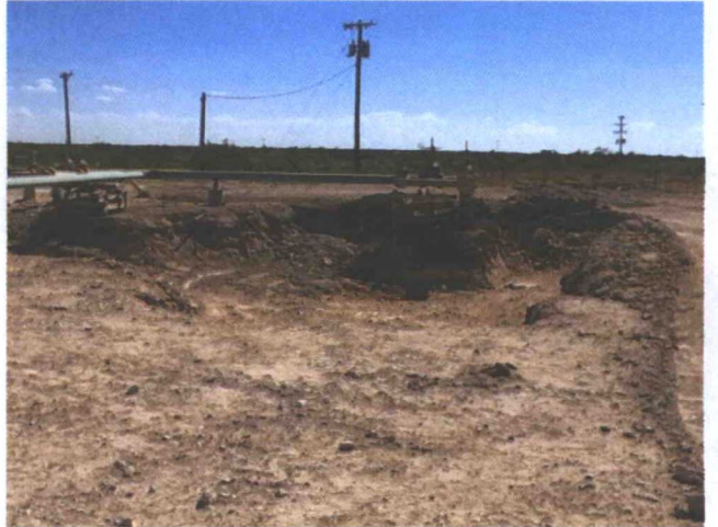
18. Test Trench 1 North wall horizontal excavation
