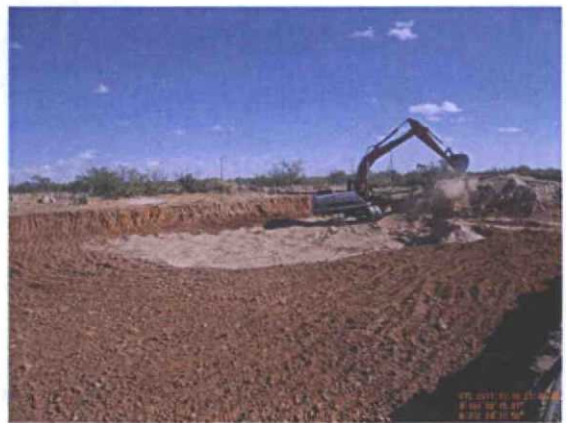
East side, placing sand pad over caliche, facing Southeast 10/10/11
