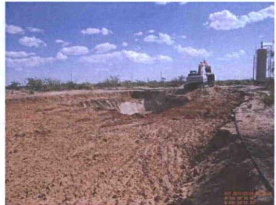
East side, 21 ft excavation complete, facing south 9/26/11
