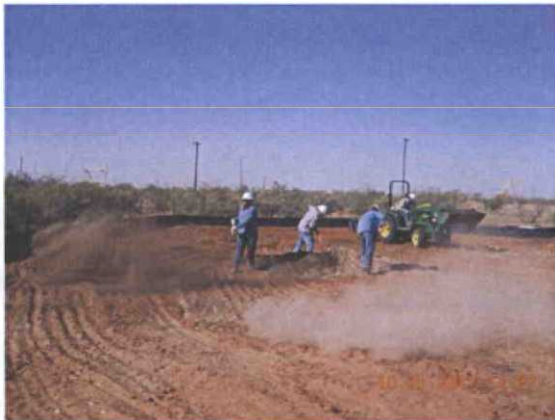
West side, adding soil amendments, facing north 10/21/11
