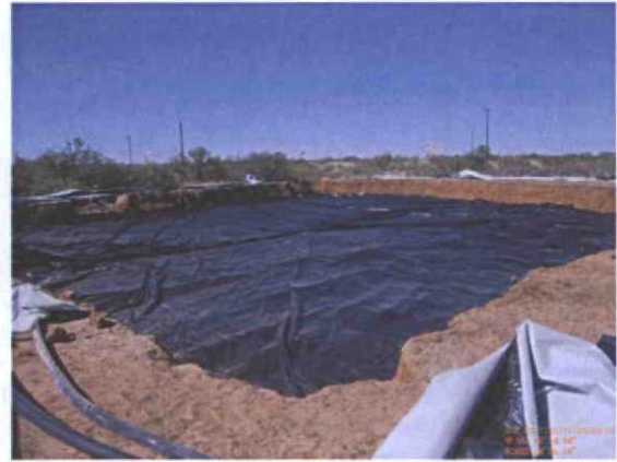
East side, liner installed at 5 ft, facing northwest 10/11/11
