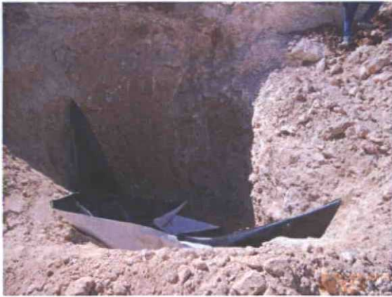
West side, installing liner over clay layer, facing west 10/6/11
