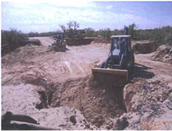
West side, backfilling 21 ft excavations, facing south 10/11/11
