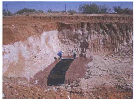
East side, clay layer completed in 21 ft excavation, facing northeast 10/6/11
