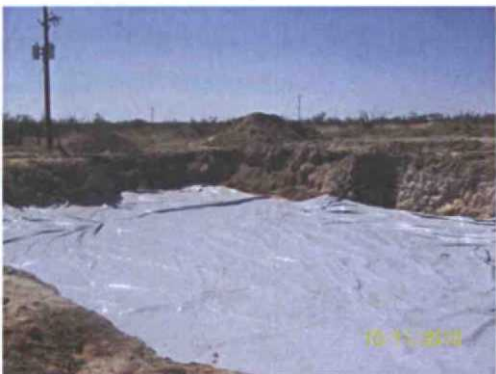
48x55-ft, 20-mil reinforced liner installed at 4.5' bgs, facing southwest 10/11/2010
