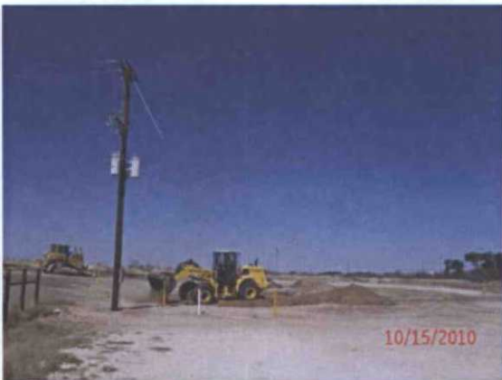
backfilling with top soil, facing north 10/15/2010
