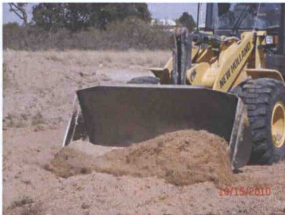
spreading amendments and contouring site 10/15/2010
