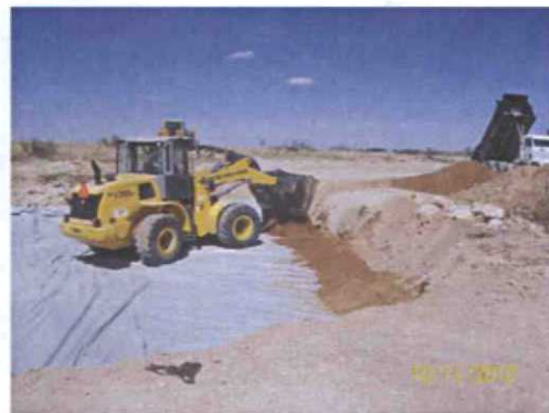
padding the liner with blow sand, facing north 10/11/2010
