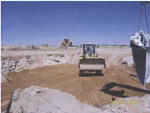
padding the site with 6 inches of blow sand, facing north 10/11/2010
