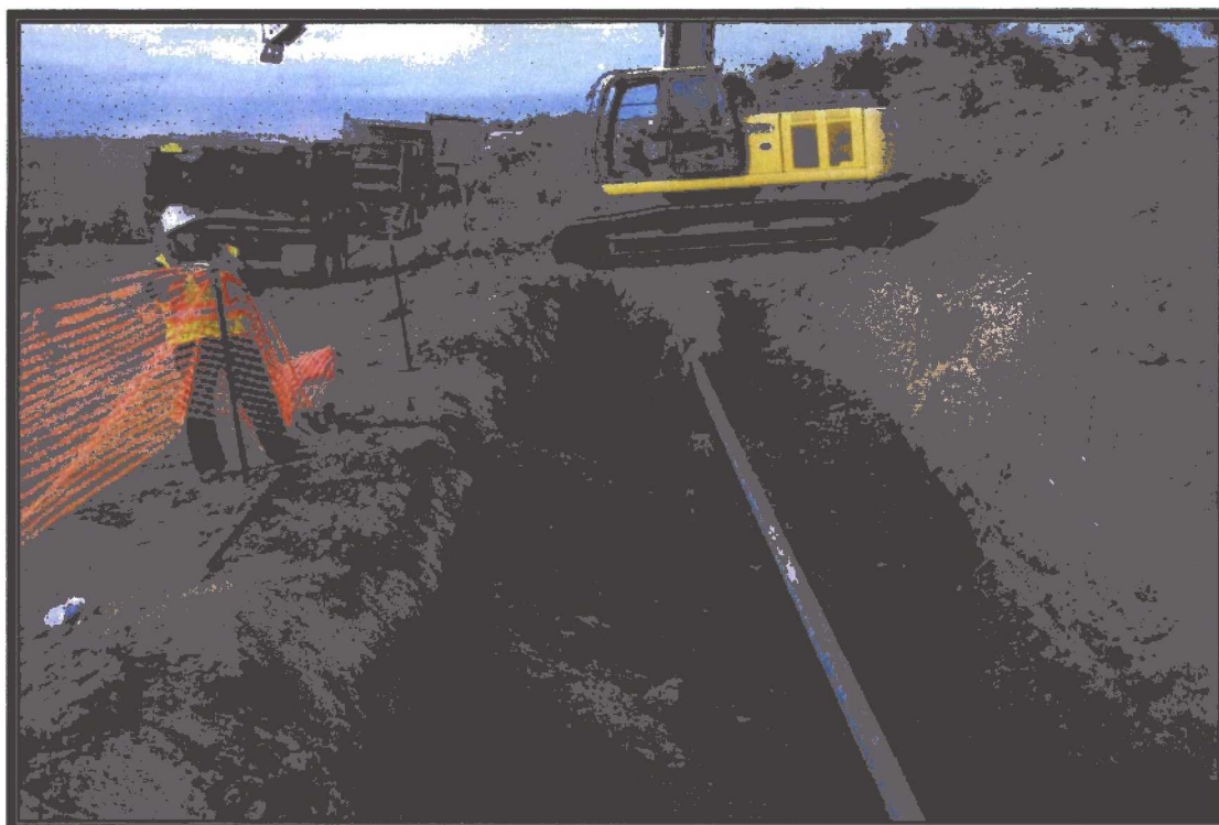
Photo 8: View of backfilling activities after the completion of excavation activities.
