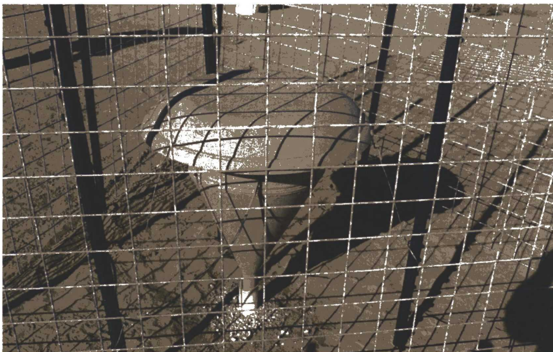
Photo 4: View of the soil vapor extraction ventilation system.
