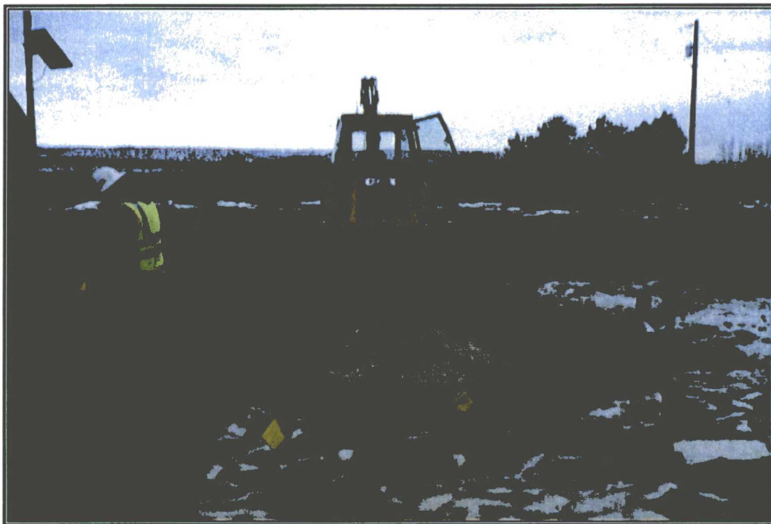
Photo 5: View of backfilling activities after completion of excavation activities and meter tube removal.
