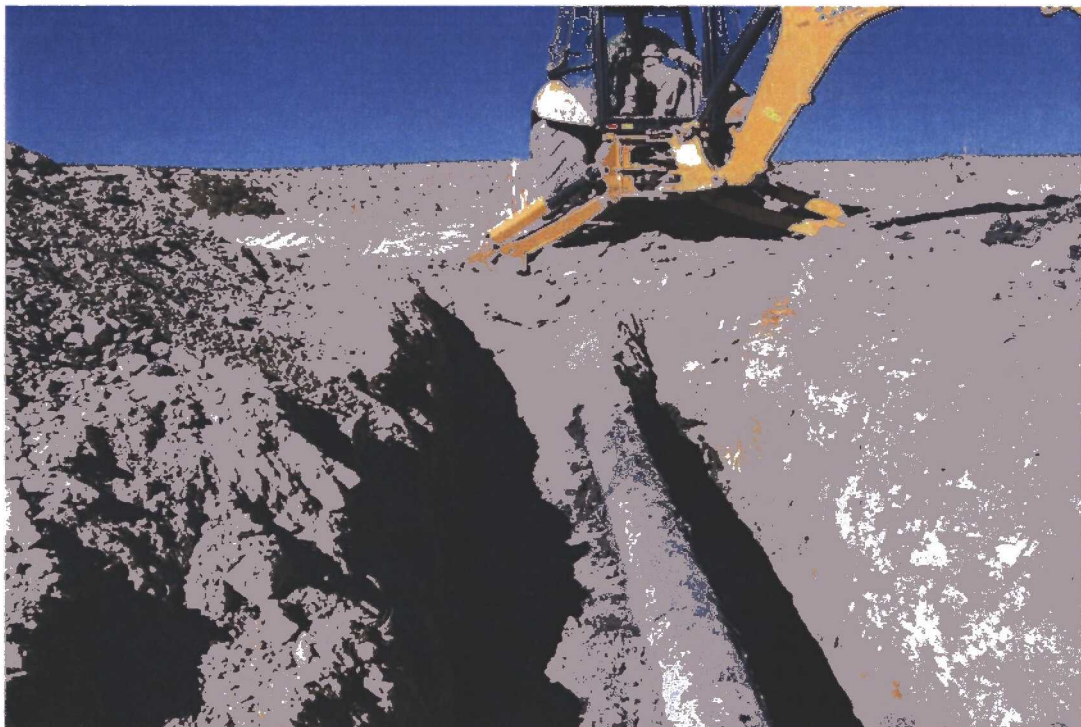
Photo 2: View of the excavation around the pipeline.
