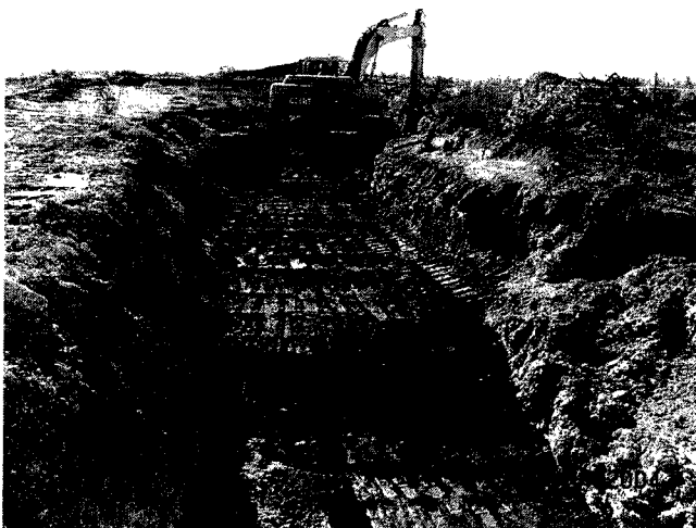
Photograph #5- Initial compaction of clay liner in eastern portion of excavation, looking westerly.
