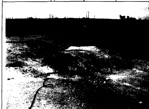
Additional excavation conducted on 5-26-07 after tank was removed to reach elevated areas from the spill
