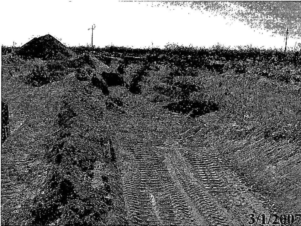
Photograph #6 – Looking west at excavation and benching of sidewalls.
