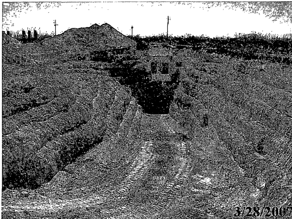
Photograph #8 – Looking west at excavation and benching of sidewalls.
