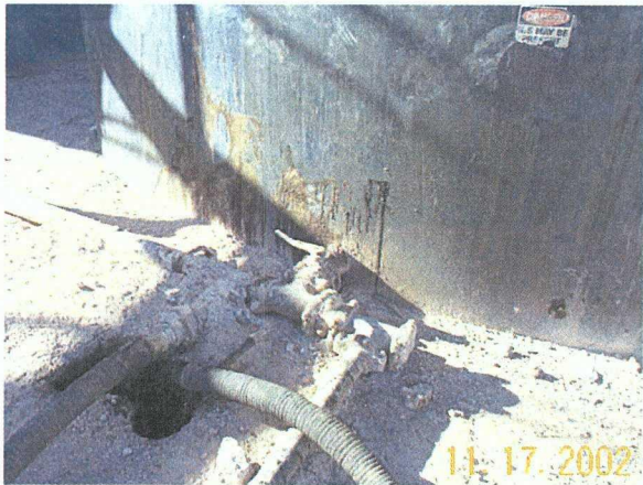
Photo 2. Sump appears to be damaged.
