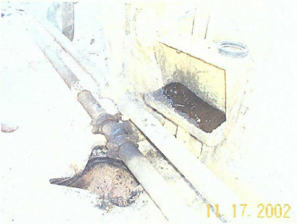
Photo 3. Sump appears to be damaged.
