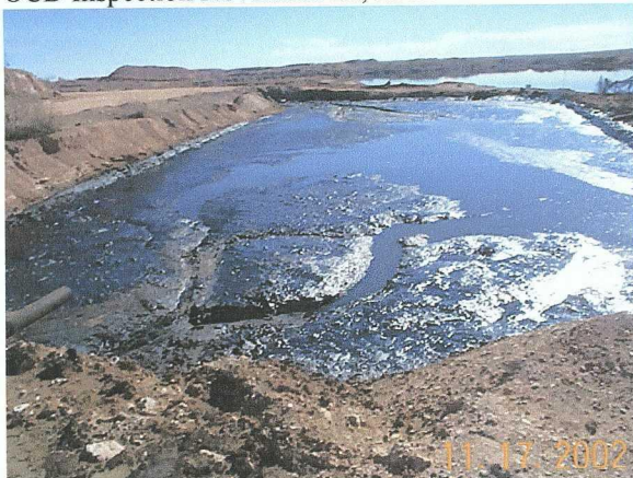
Photo 13. Decommissioning Pit 5. draining water and skimming oil.
