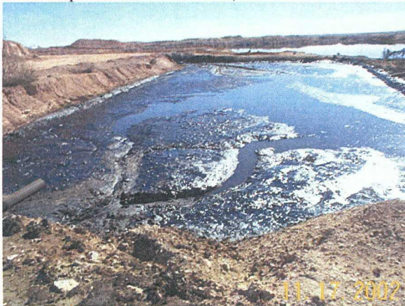
Photo 13. Decommissioning Pit 5, draining water and skimming oil.
