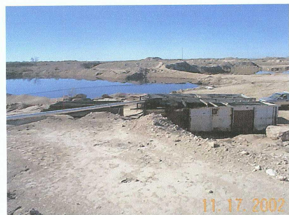
Photo 12. Produced water steal pit system below the produced water receiving tanks. Pits are screened.
