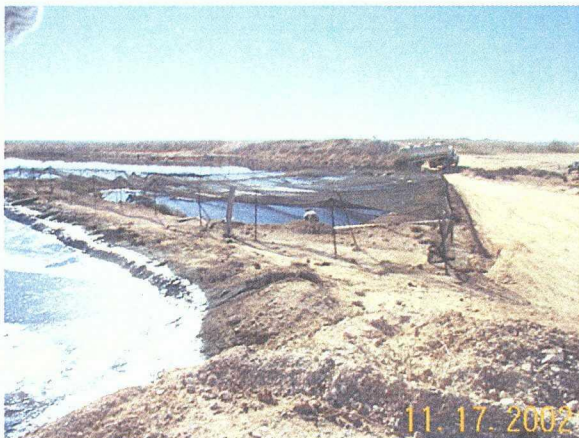
Photo 14. Decommissioning Pit 5, draining water and skimming oil.
