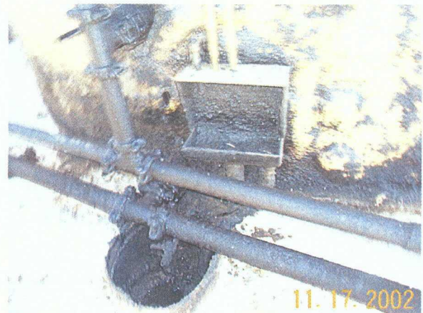
Photo 5. Sump in place below a valve that shows signs of leaks. Sump was empty.
