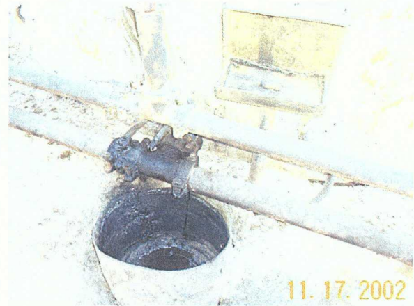
Photo 4. Leaking valve. Catchment in place and empty.
