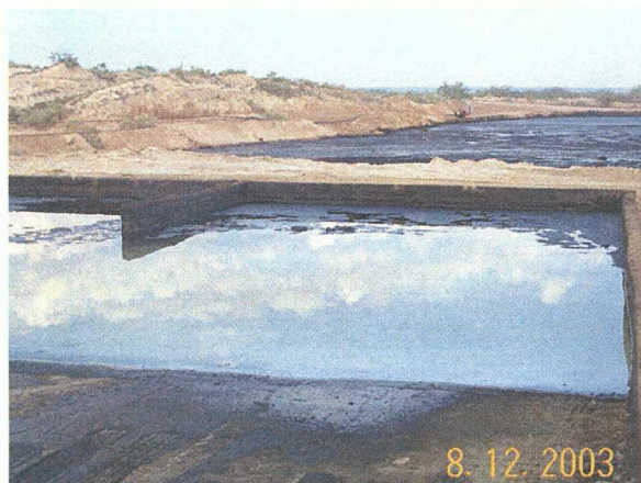
Photo 7: Concrete lined Truck washout pit. Grate is missing. Looking west toward Pond 4.
