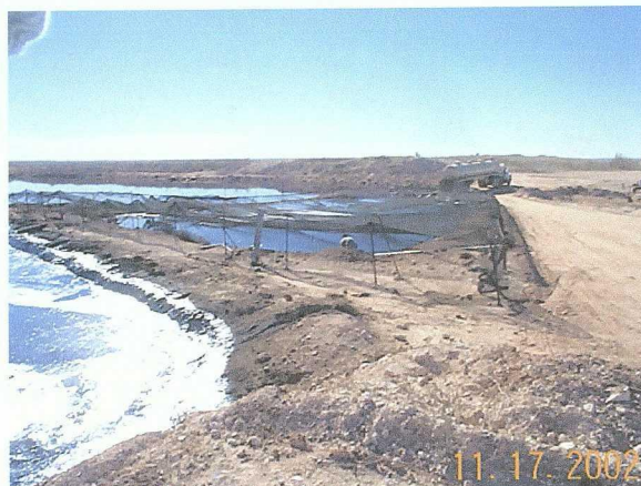
Photo 14. Decommissioning Pit 5. draining water and skimming oil.
