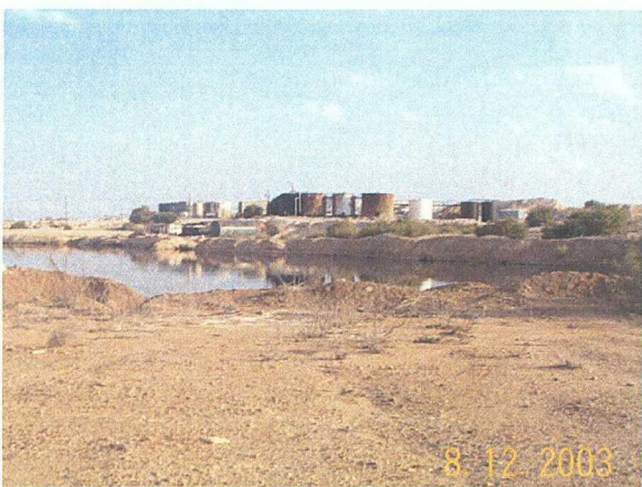
Photo 15: Pond 1 was oil free. Treating plant is on the hill and the new skim tanks that are replacing the skim pits at pit 5 are below the hilltop.
