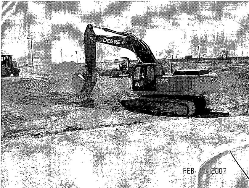
Placing final backfill layer into the right-of-way
