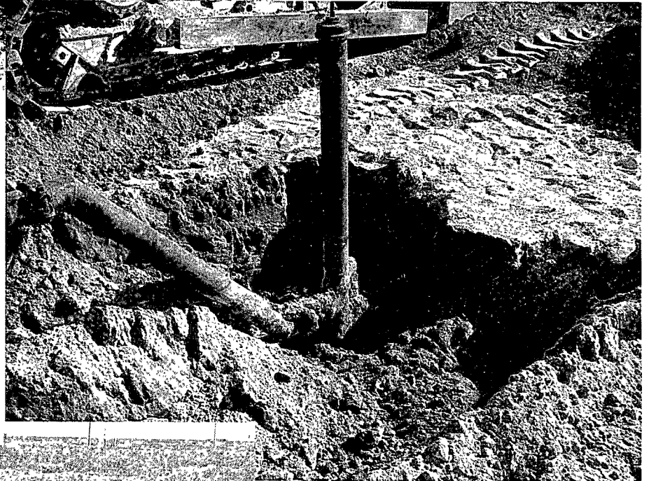
Riser near oil sump exposed. Pipes were eventually removed.
