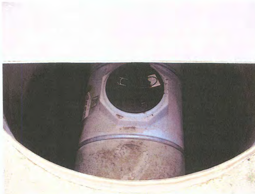
Figure 9: TK-6 325 Gallon Poly Waste Oil Tank in Fiberglass Vault
