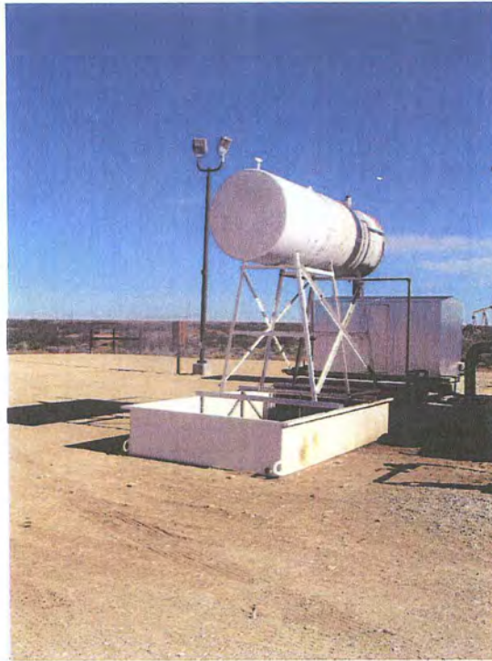
Figure 7: 1000 Gallon Steel Lubrication Oil Tank TK-5 and 1100 Gallon Steel Secondary Containment (note vault for TK-6 by lower right corner of TK-5 containment).
