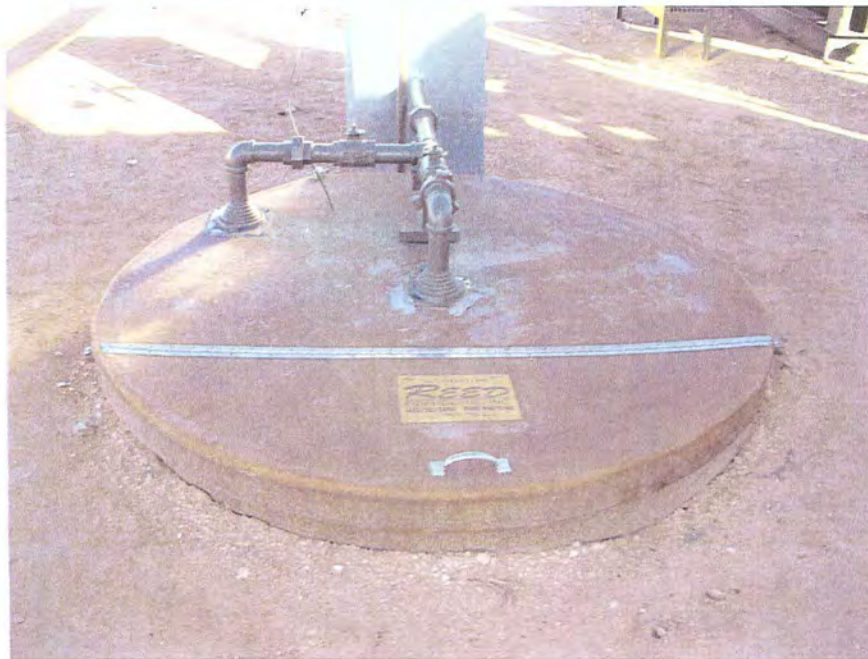
Figure 8: Top Cover of Double Walled Fiberglass Vault Holding Waste Oil Tank TK-6
