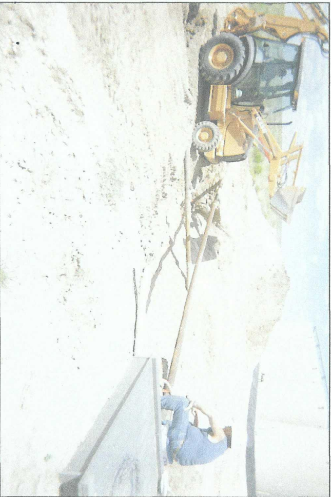
backfilling excavation (with new junction box)
