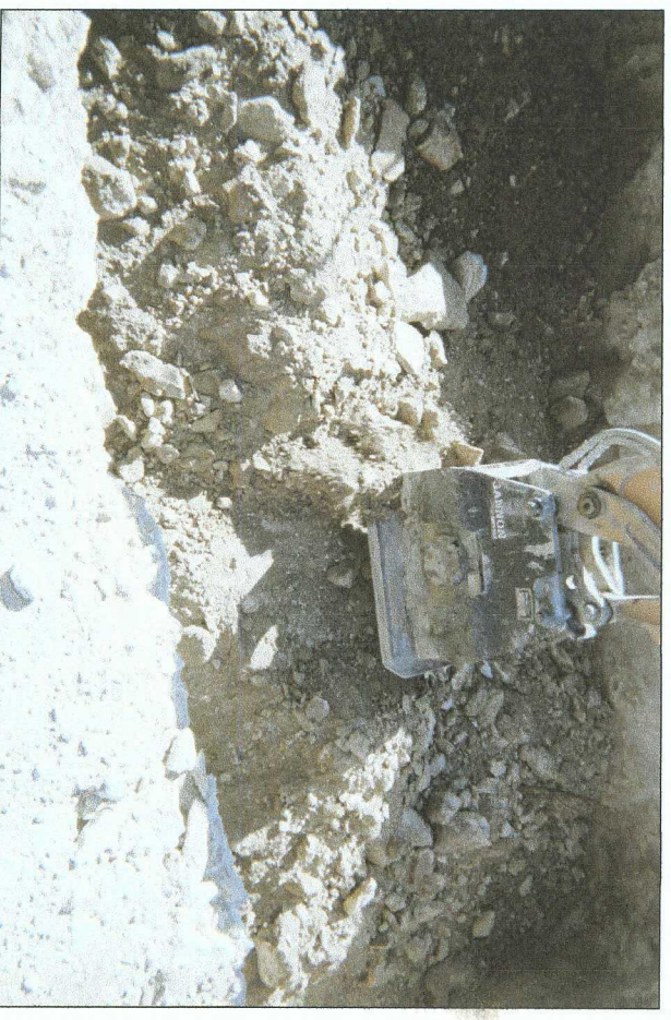
compacting backfill 2/15/06
