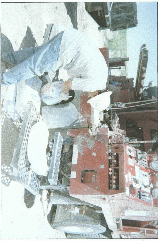
plugging soil bore with bentonite
