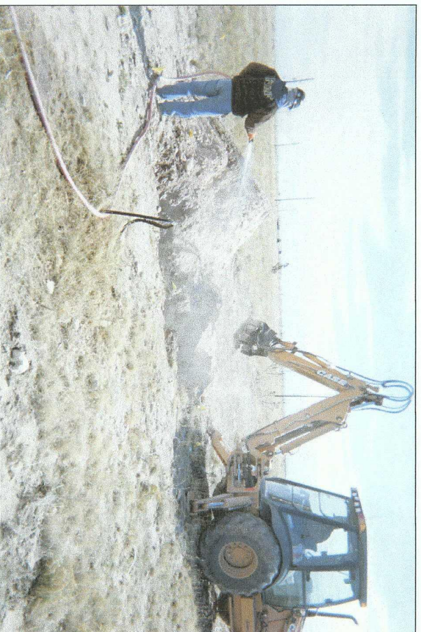
backfilling delineation trench
