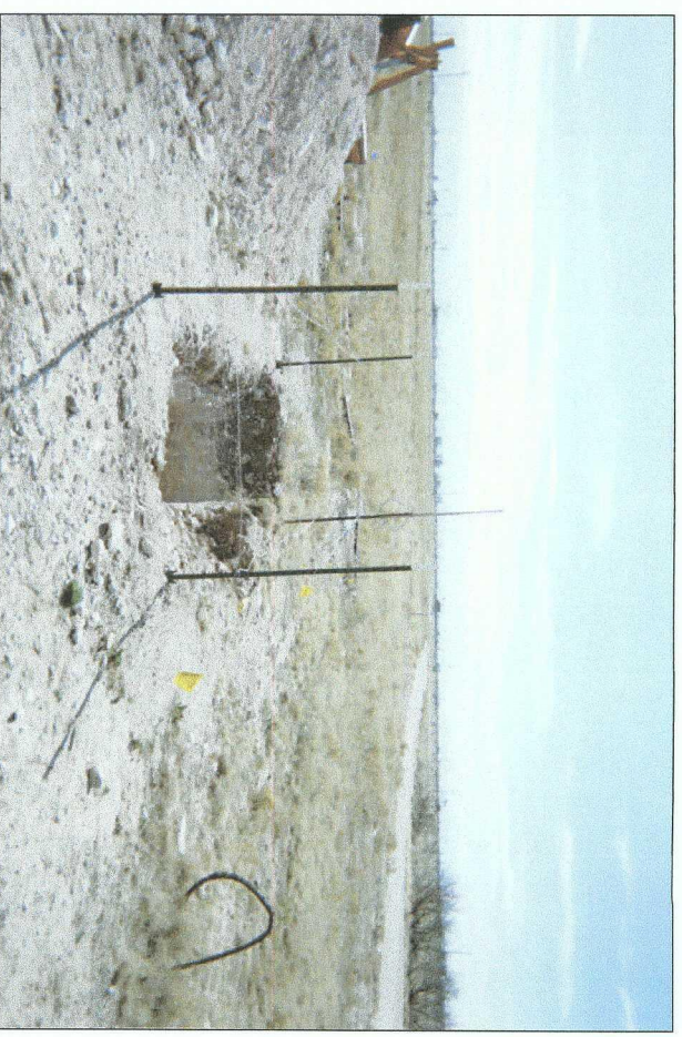
delineation trench to 12 ft BGS make with trackhoe
