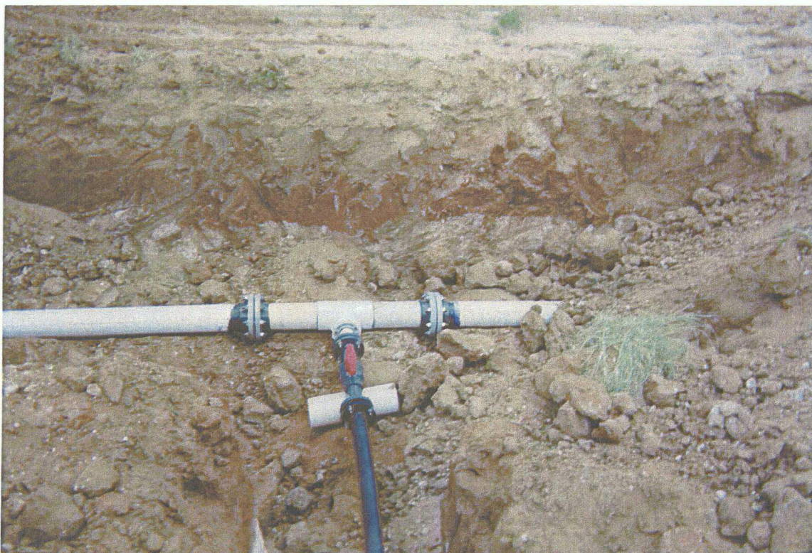
11. Plumbing for new junction box.
