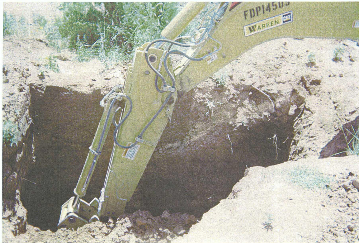
3. Excavation of the old junction box.
