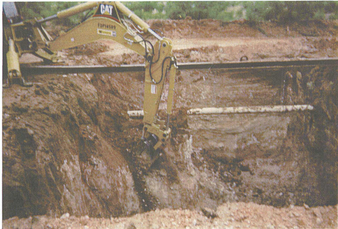
5. Excavation of the old junction box.
