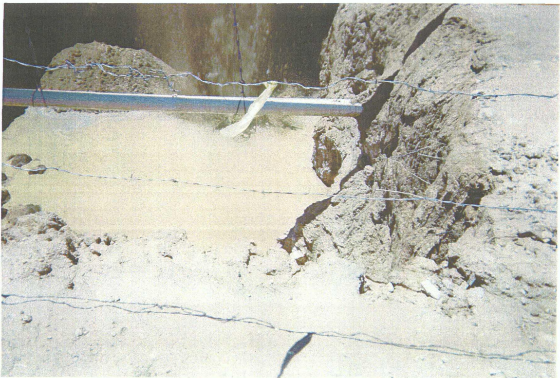
6. Backfilling of the old junction box.
