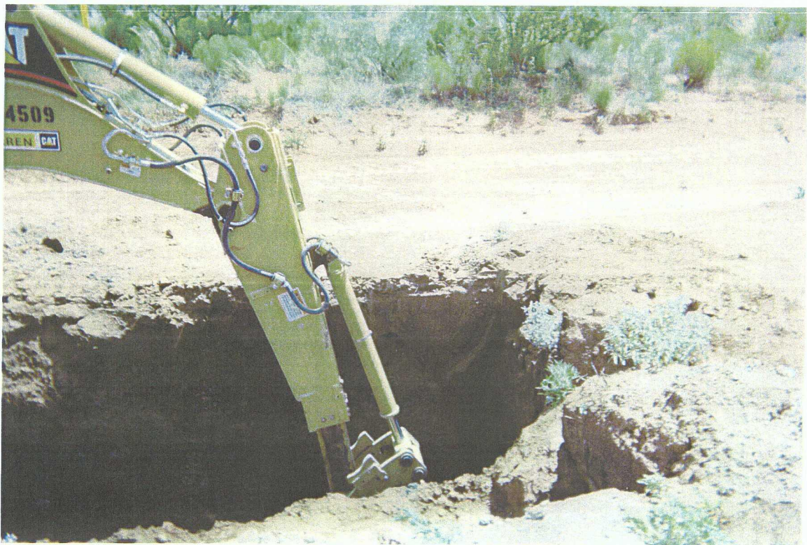
4. Excavation of the old junction box.
