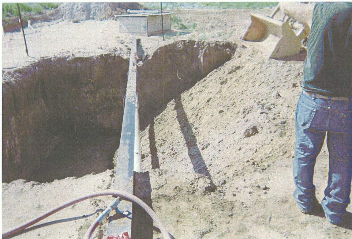
7. Backfilling of old junction box.
