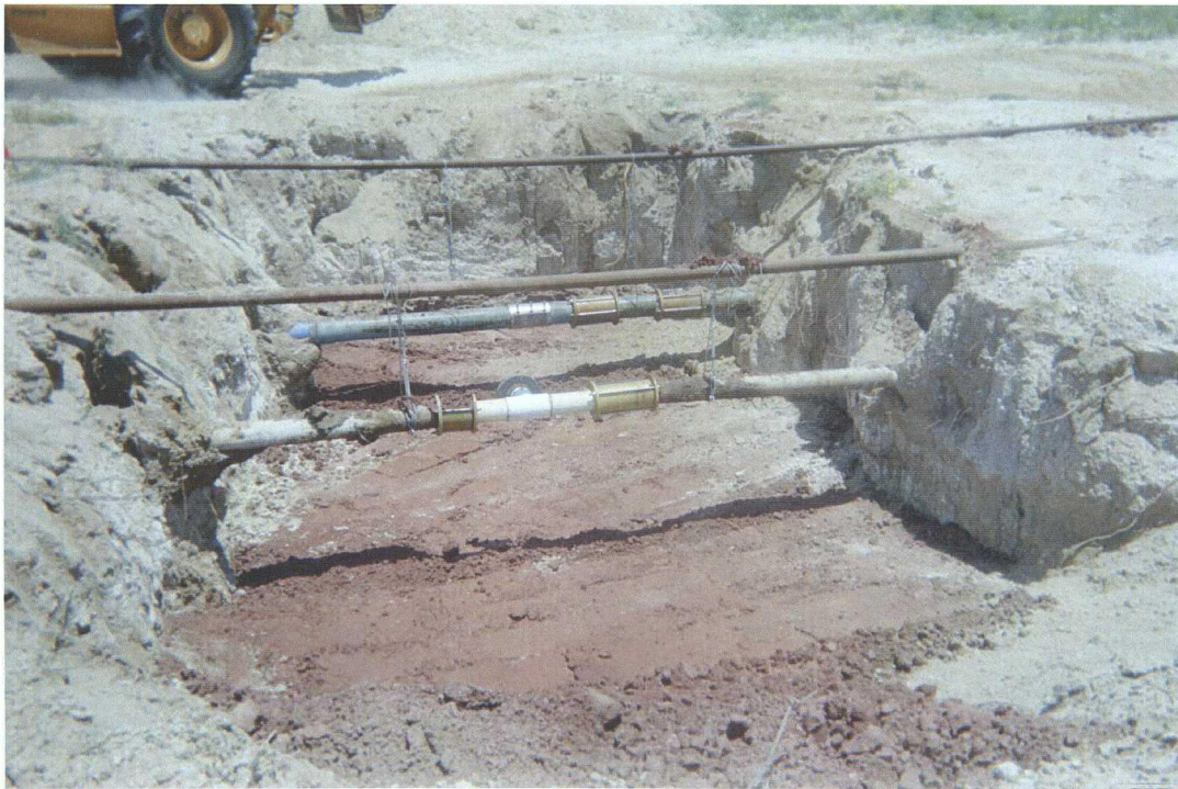
View facing east showing compacted clay barrier at 5 ft below ground surface (07-07-2004).
