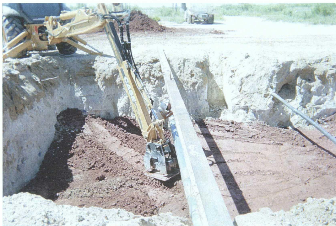
View facing south showing compaction of clay barrier at 5 ft below ground surface (07-14-2004).
