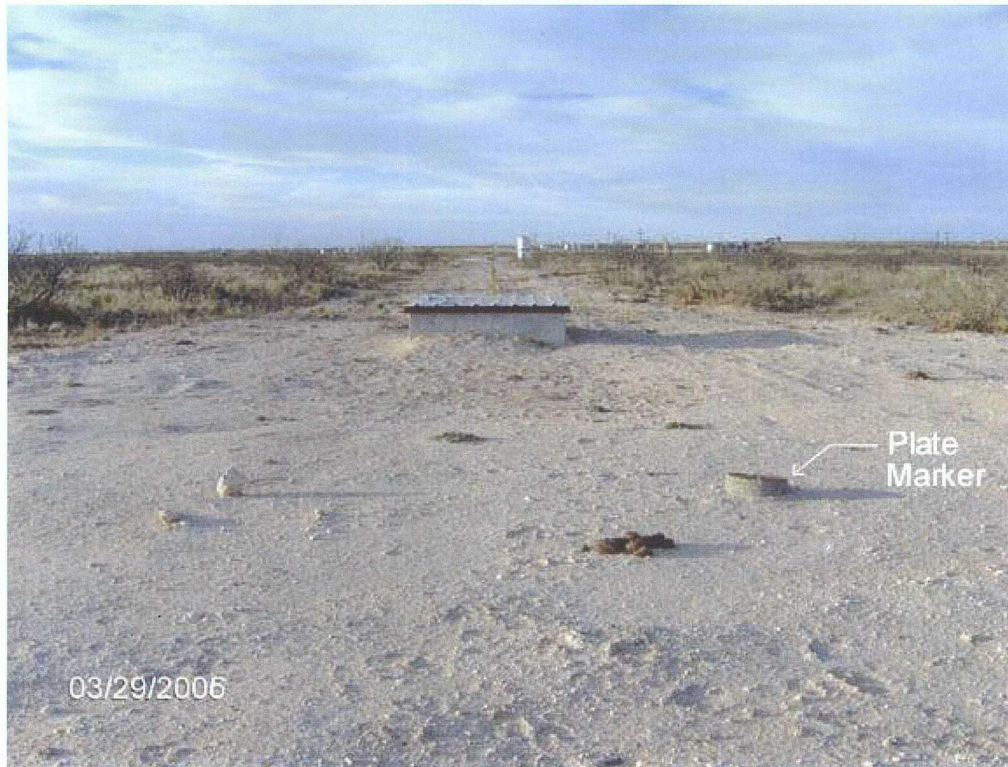
Recent view facing north showing plate marker over former vent location in foreground and new junction box in background (03-29-2006).
