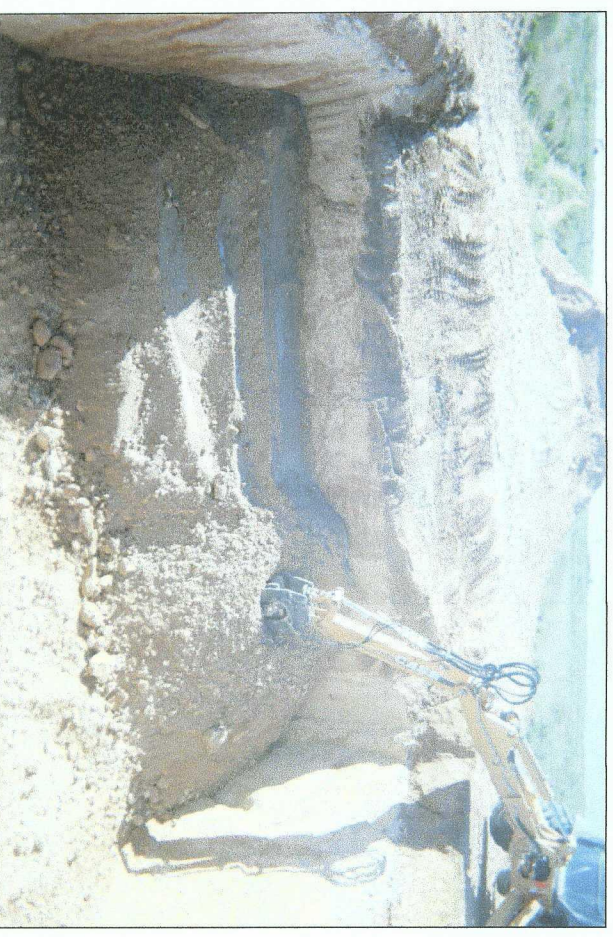
backfilling final 30 x 30 x 12-ft-deep excavation
