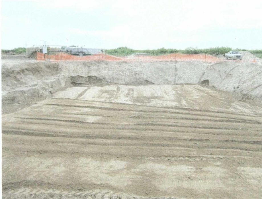
Photo 5 - Excavation being backfilled with clay barrier from to 5.5 to 7 ft. bgs (5/14/07).
