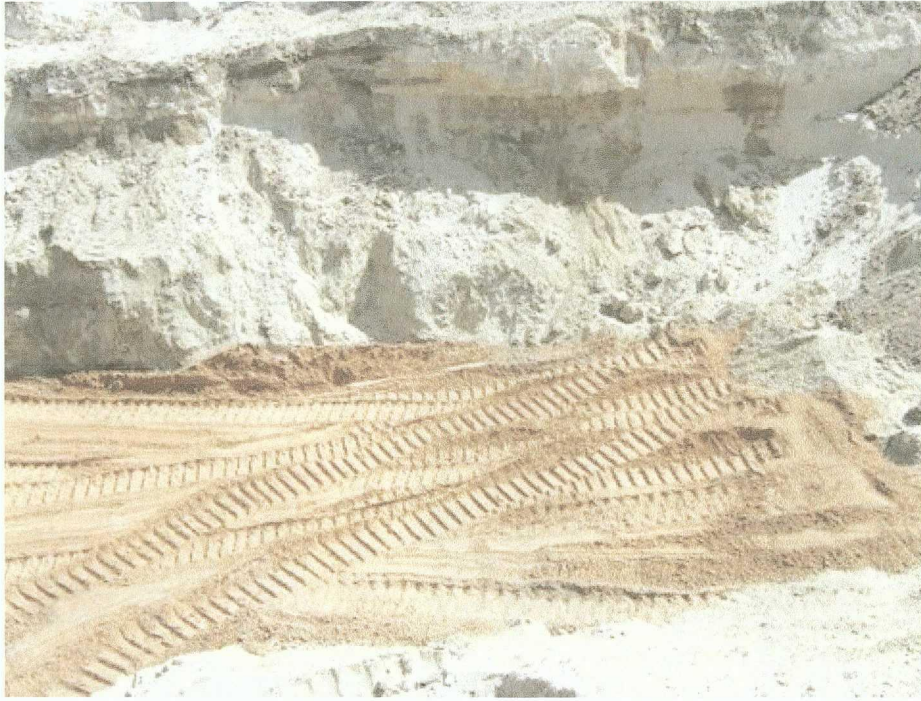
Photo 3- Clean soil being backfilled into excavation (4/12/07).
