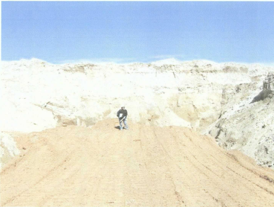
Photo 4 - Excavation backfilled to 20' bgs with clean soil (4/16/07).
