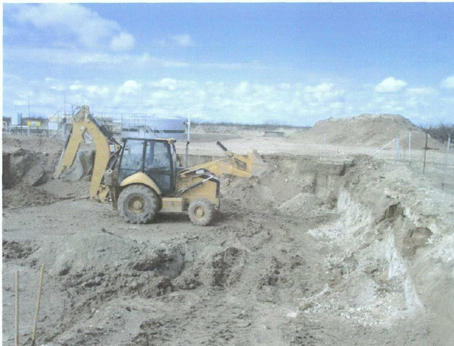
Photo 1- Excavation of pit at former tank locations (4/9/07).
