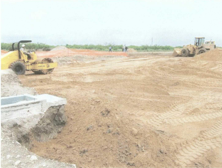
Photo 7- Clean topsoil backfilled over clay barrier (5/17/07).
