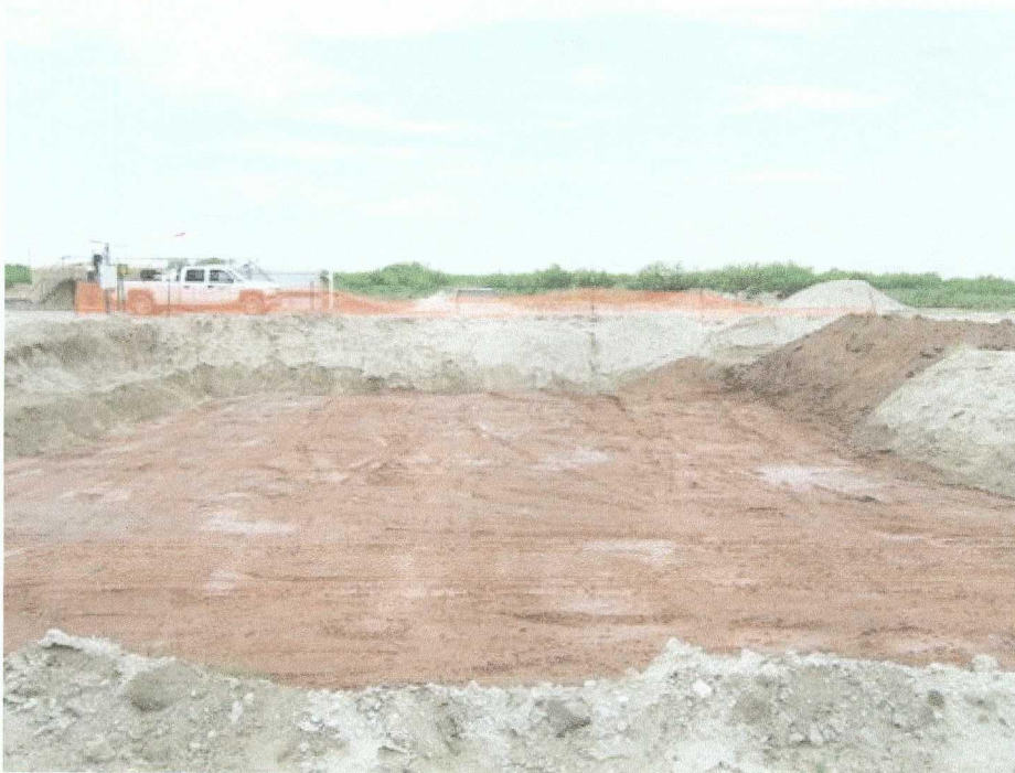
Photo 6 - Top of clay barrier just prior to compaction test (5/15/07).
