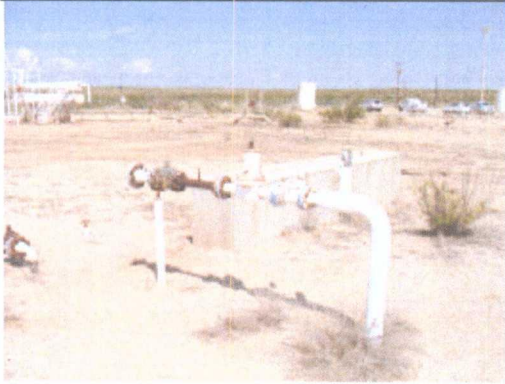
Photo 13 : Remaining protruding underground conduit.
