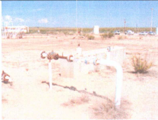
Photo 13 : Remaining protruding underground conduit.
