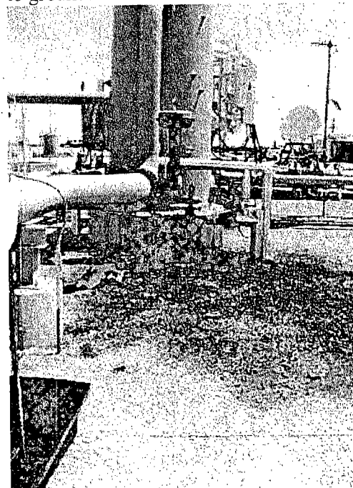
Photo 26: Sulfur unit with discharge on ground.
