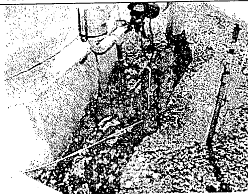
Photo 25: Sulfur unit with discharge on to ground.
