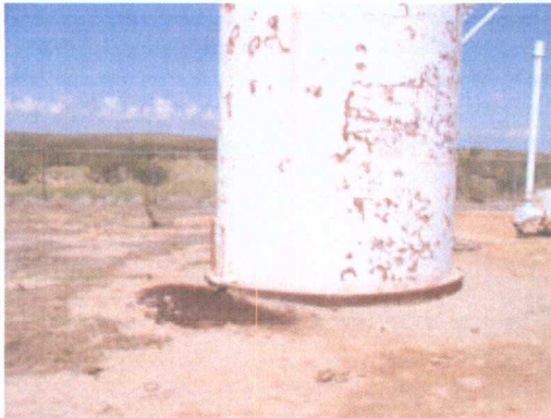
Photo 1: Used tank not in service. Leaking substance on to ground.
