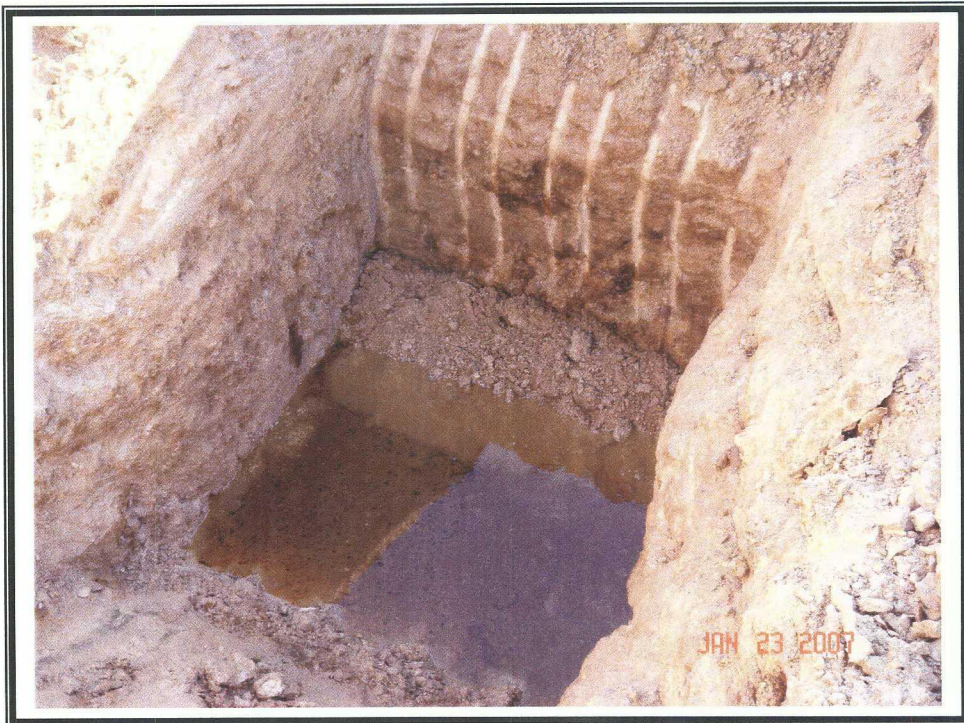
Groundwater encountered in northern floor of associated pit at Texaco Mattern Battery #26
