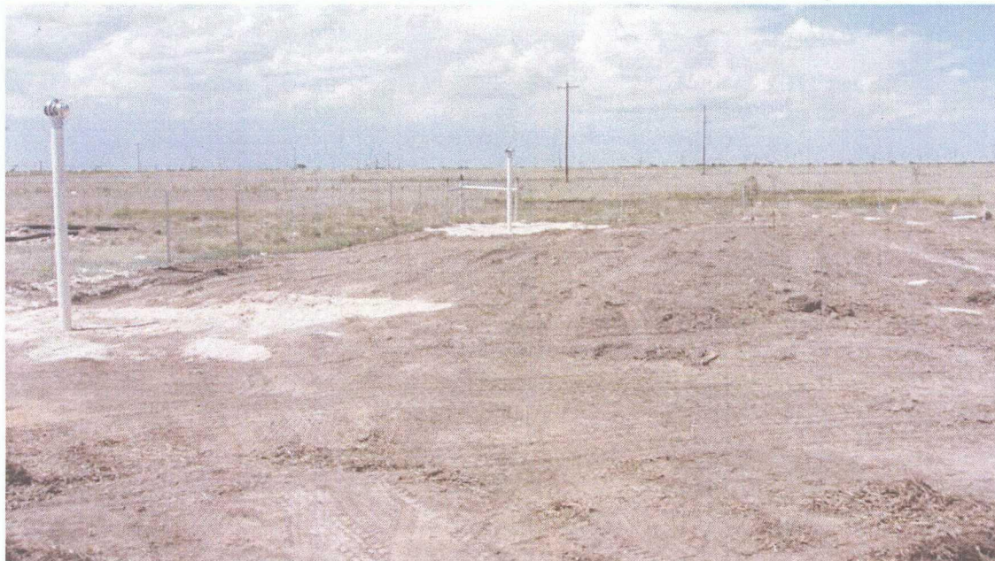
Completed soil vapor vents at G-35 (backfilled excavation visible to right of vents)
