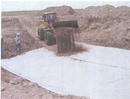
GCL at F-35, placed 7 feet below grade
