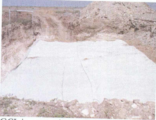
GCL in excavation at G-35, 7 feet bgs
