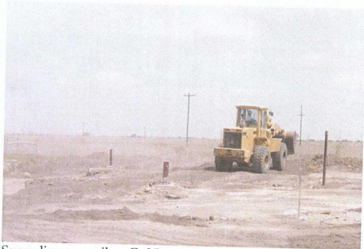
Spreading topsoil at G-35
