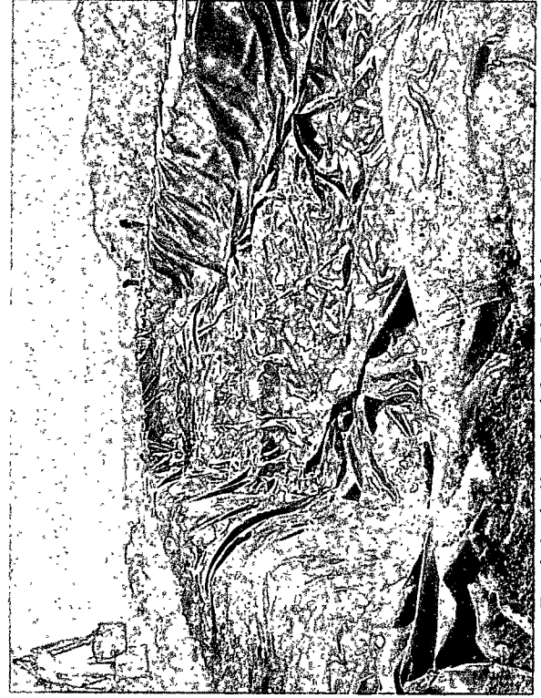
Burial pit lined with a 20 mil impervious liner.
