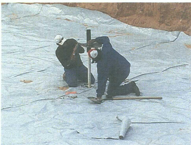
Jalmat 1 – liner being fitted with boot at base of monitor well..
