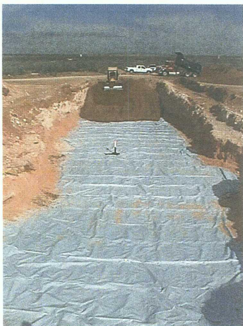
Jalmat 1 – Liner install complete and backfill over liner initiated.
