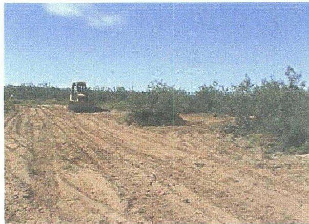
JALMAT 2 Photo from same locations as above following blending of soils to 2 ft bgs.
