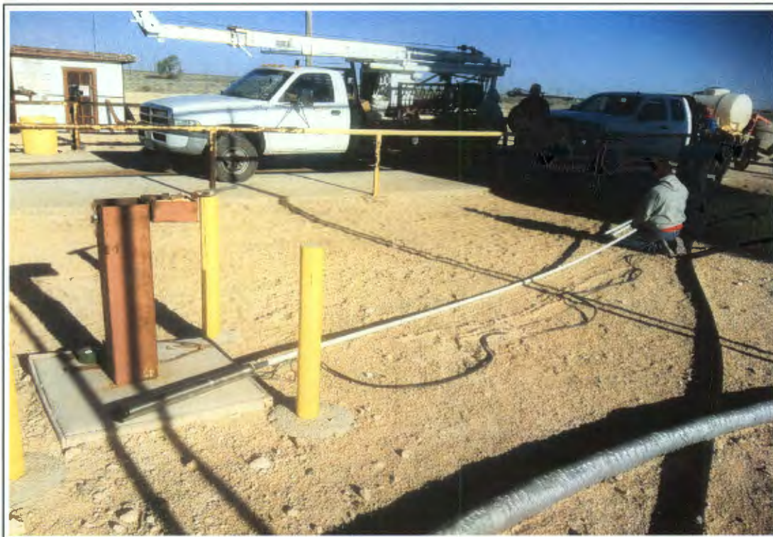
5. Grundfos submersible pump and drop pipe connection
