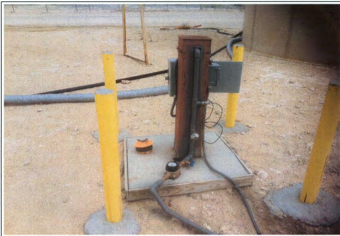
8. Completed installation for RW-1
