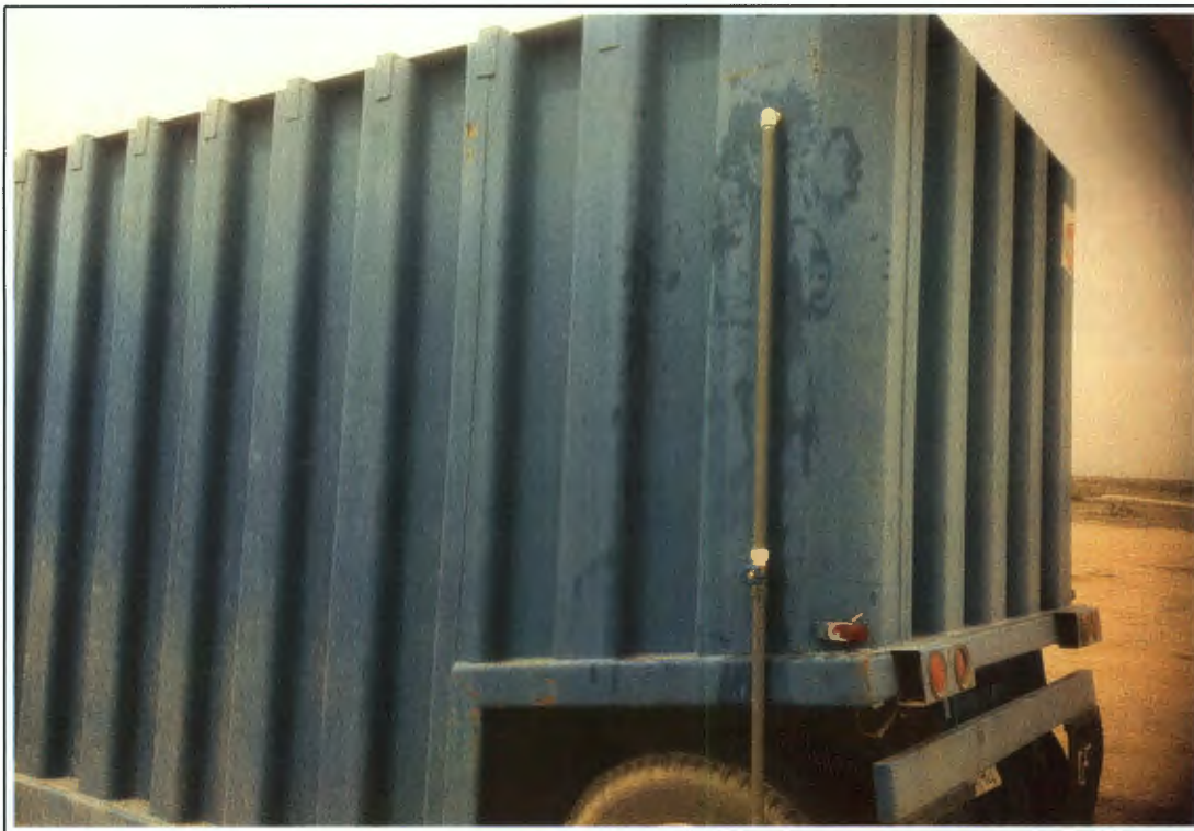
7. Termination of conveyance piping into frac tank for RW-2
