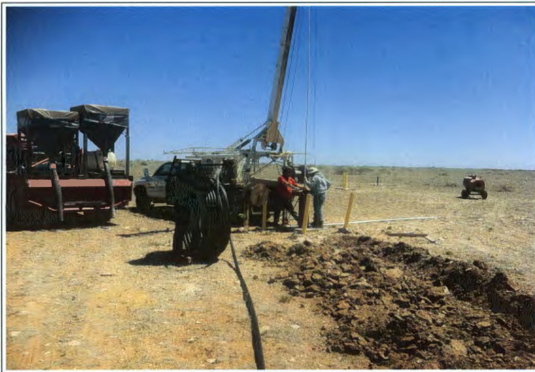
3. Installation of conveyance piping and pump at RW-2
