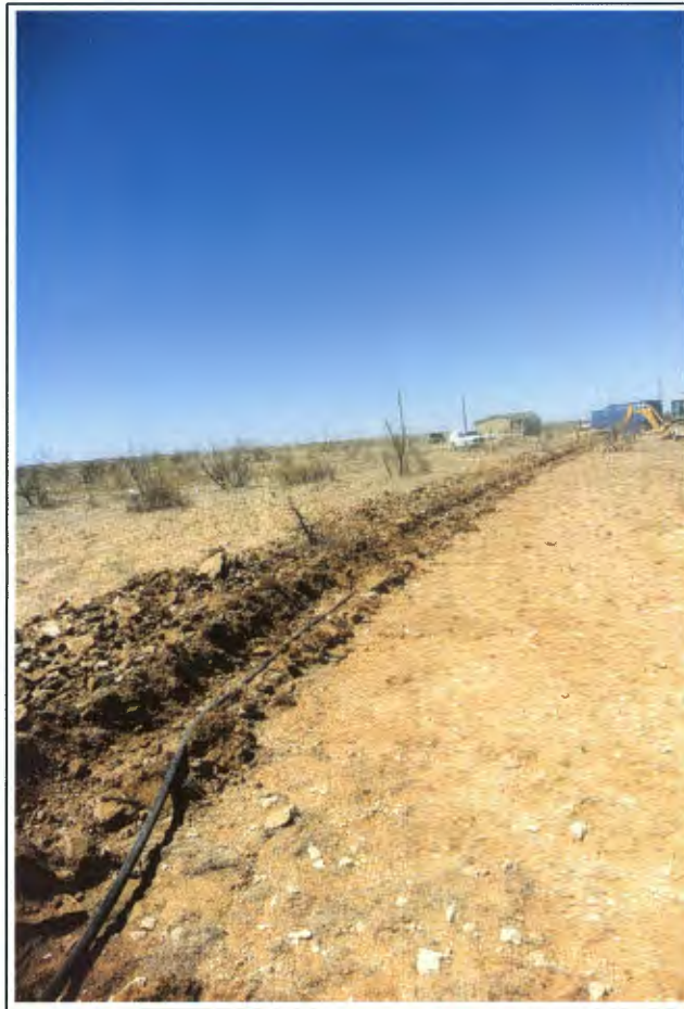
2. Installation of conveyance piping from RW-2
