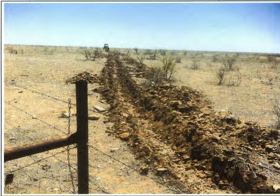
1. Trenching for conveyance piping installation for RW-2
