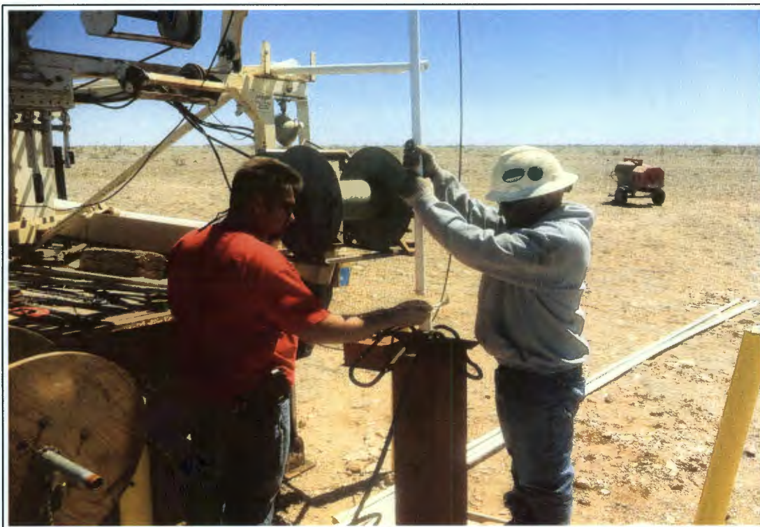
4. Making drop pipe connection during installation of pump in RW-2
