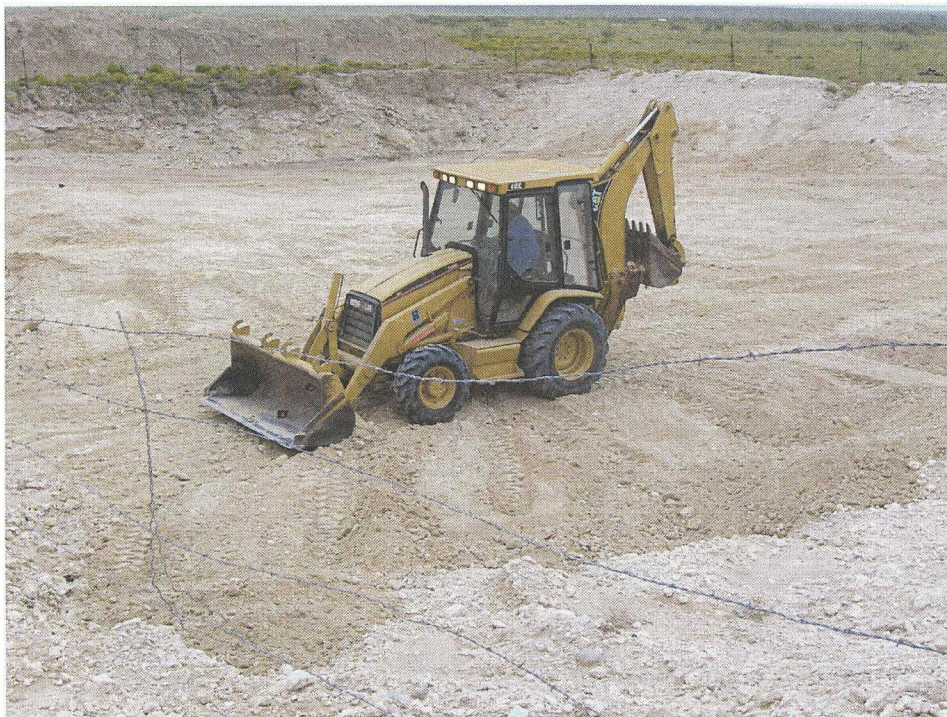
SMOOTHING EXCAVATED BOTTOM – PREPARING TO DRILL
