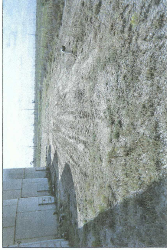
site backfilled with 12 yds 3 imported fill
