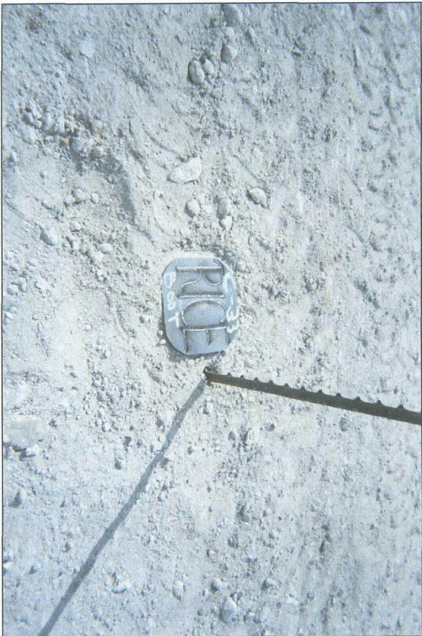
identification plate at surface of backfilled site marking former junction 10/11/2007
