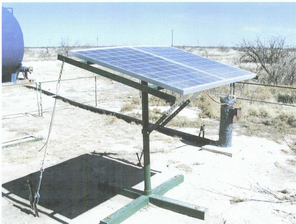
Figure 5 – Photograph of solar-powered groundwater recovery system.
