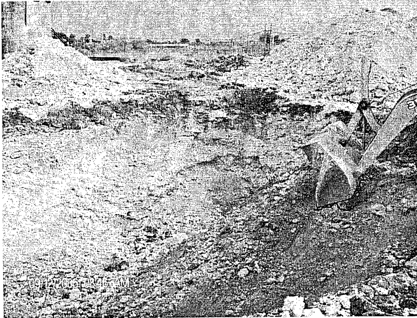
Figure 3: Backfilling excavation with blended soil
