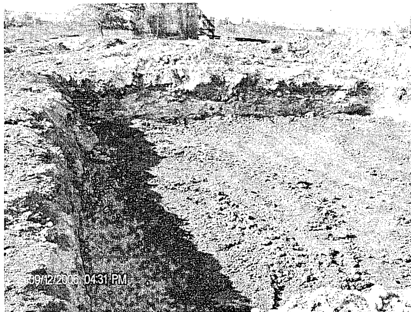
Figure 8: Clay placed in excavation
