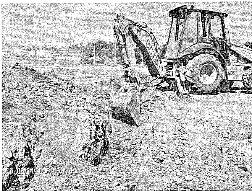
Figure 2: Digging out abandoned lines
