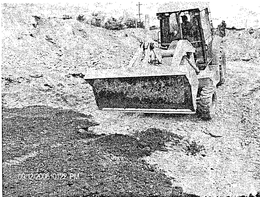
Figure 6: Compacting clay with equipment
