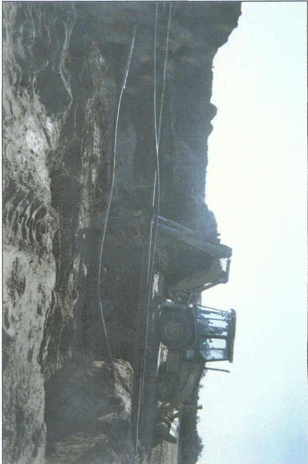
excavating 6-ft shelf around excavation 10/16/2007
